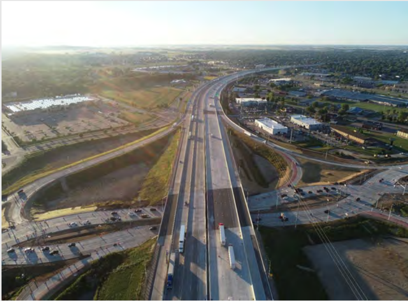
WIS 26 Interchange (looking towards Beloit)
