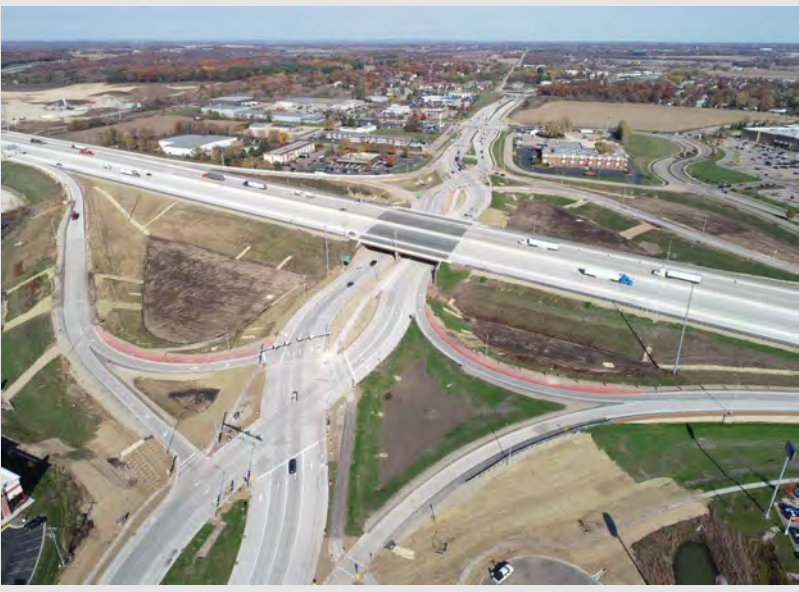
WIS 26 diverging diamond interchange (looking north)
