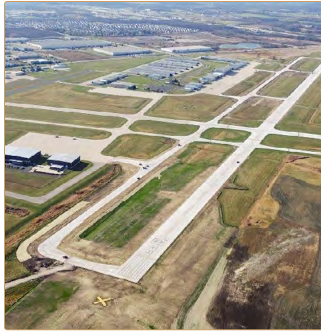
Kenosha Regional Airport runway extension
