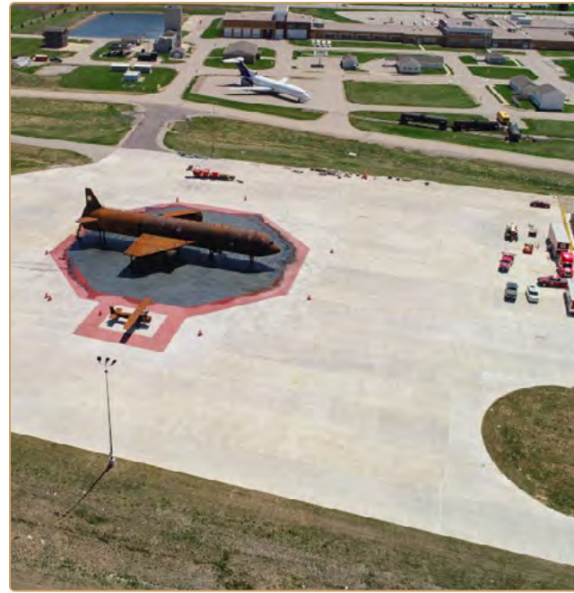
Appleton International Airport Aircraft Fire Fighting Training Facility
