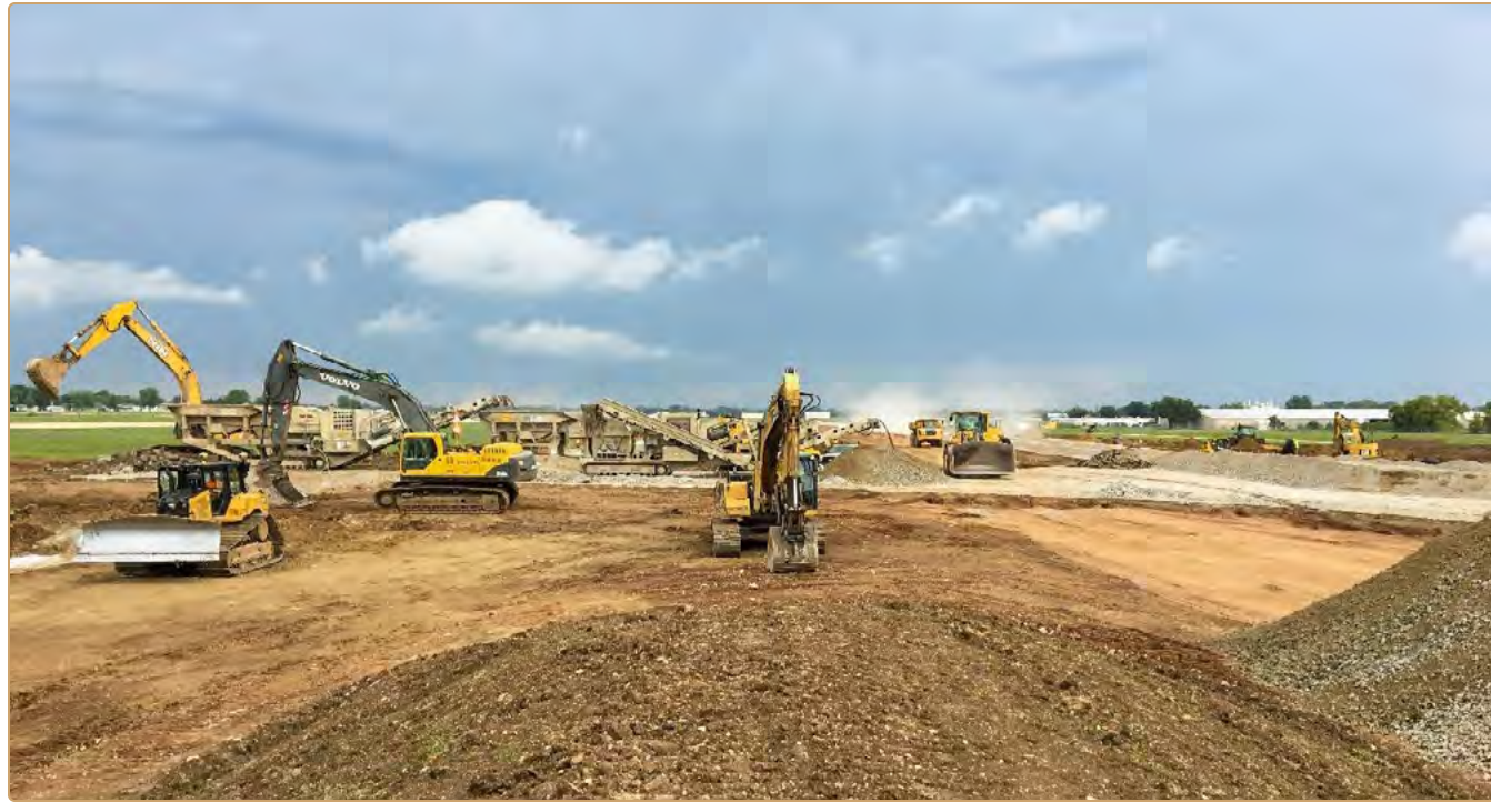
Wittman Regional Airport, taxiway construction
