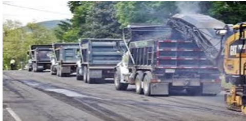
Asphalt Milling on a WisDOT Project.
