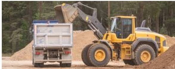
WisDOT Project Excavation.
