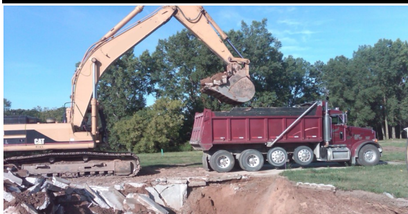
Hauling debris off a WisDOT project
