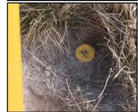
Figure 4. ROW monument with yellow cap and yellow plastic post with sign nearby. Posts may be metal too.
