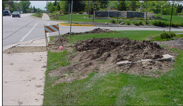
Figure 4: Examples of Improper ROW Restoration
