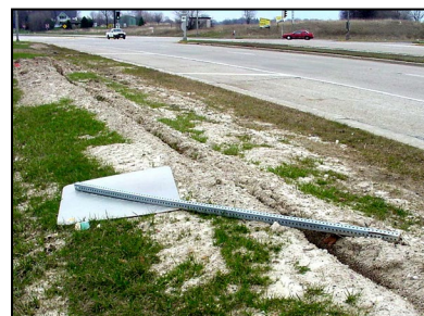
Figure 1: Improper Sign Removal
