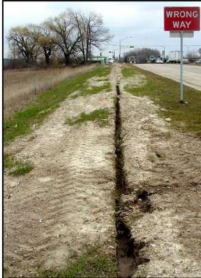
Figure 4: Examples of Improper ROW Restoration
