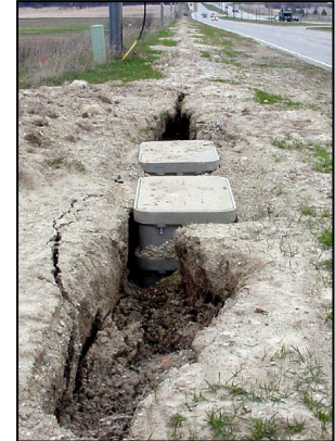
Figure 4: Examples of Improper ROW Restoration
