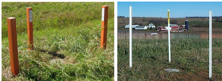
Figure 5. Orange guard or white witness posts surround a typical geodetic survey control station installation. Some of these monuments may have only 1 or 2 posts.
