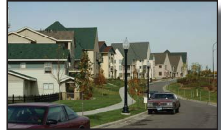
Roads and sidewalks
