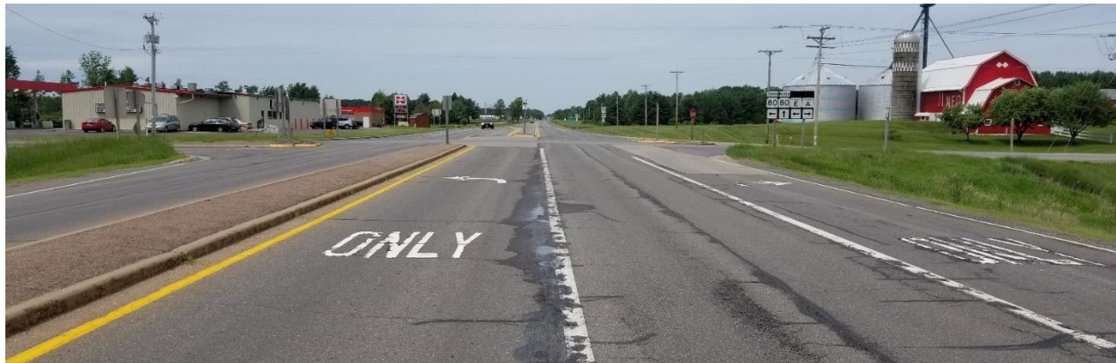
Figure 2: View approaching the WIS 73/WIS 80/Wood County A intersection traveling west on WIS 73
