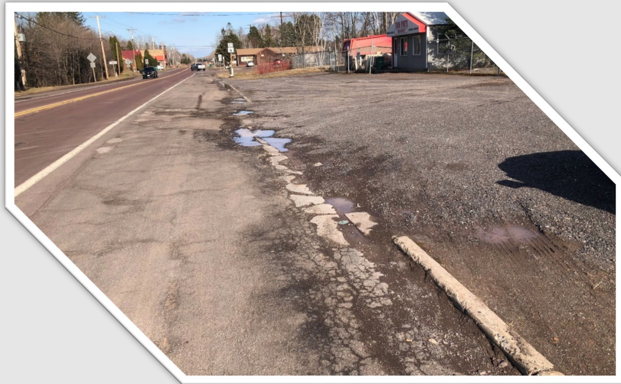
Curb and gutter in Oliver
