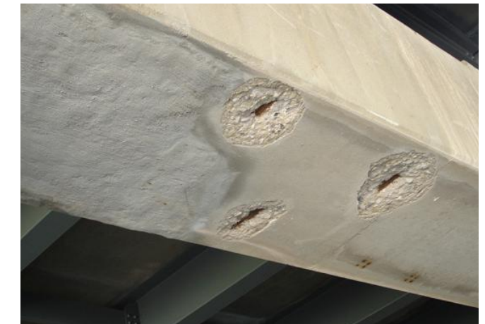
I-94 bridge over 32nd Street
