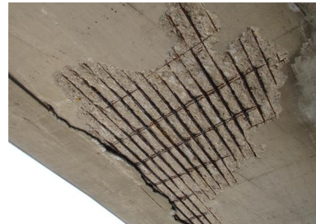
Underside of I-94 bridge over Yount Drive
