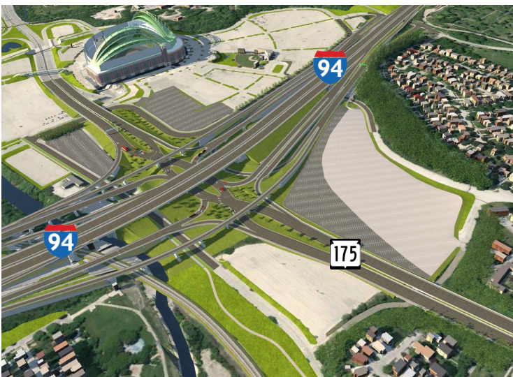
Diverging Diamond Interchange
