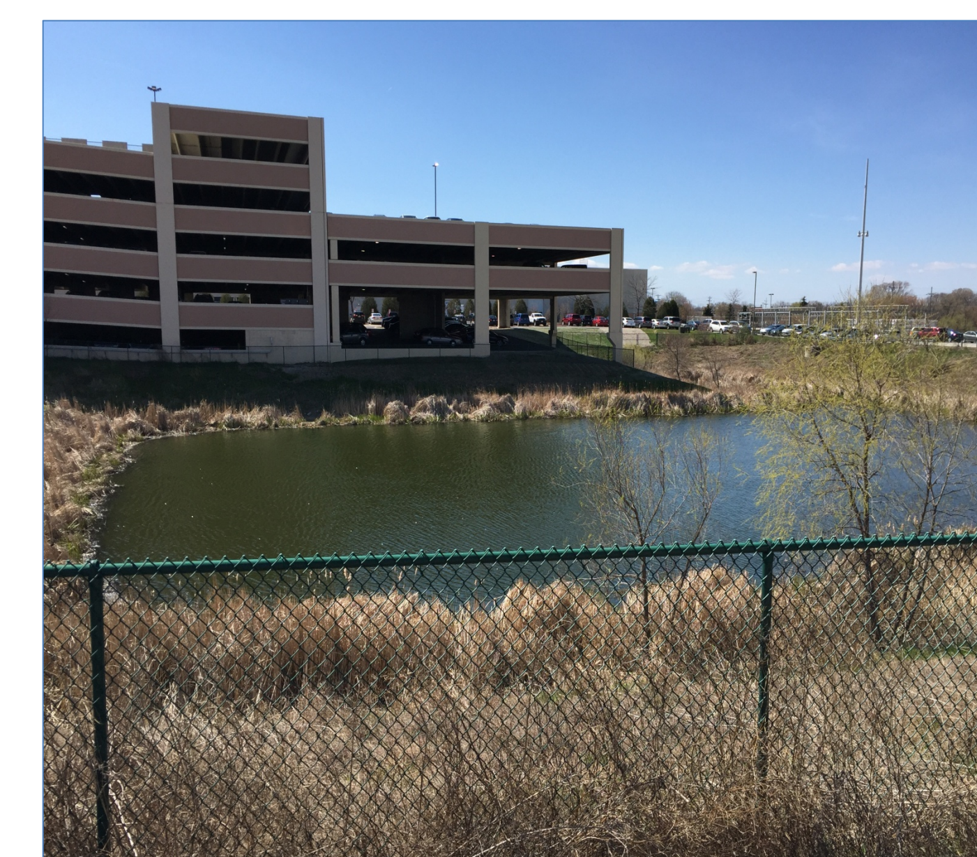
Stormwater Detention Pond
