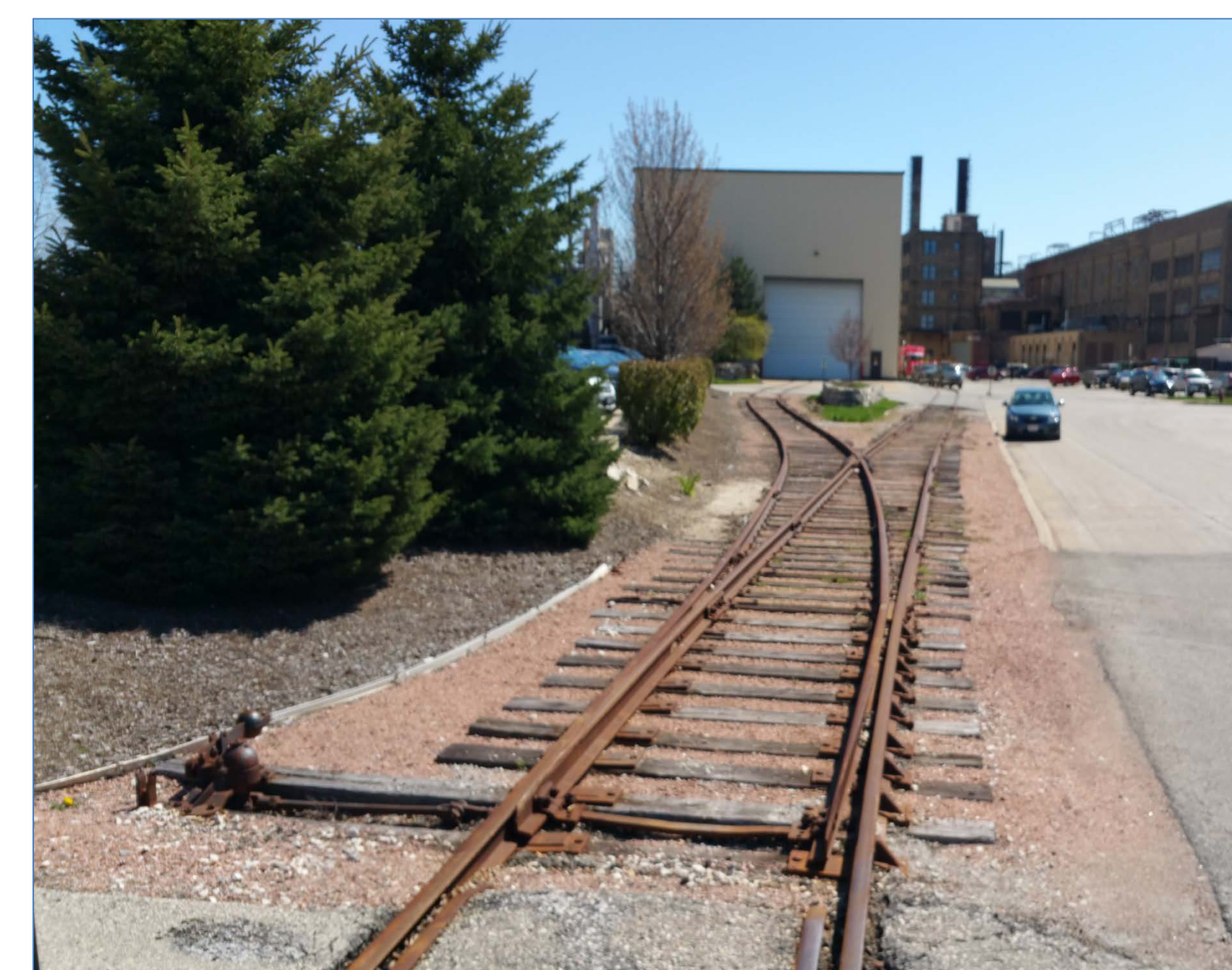
Active Railroad Spur Switch
