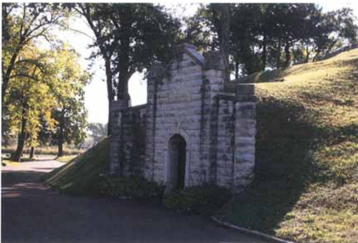
Photograph 12 of 23. Deuster Family Vault, view facing east.
