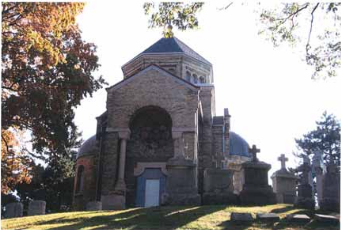
Photograph 6 of 23. Calvary Chapel, view facing east.
