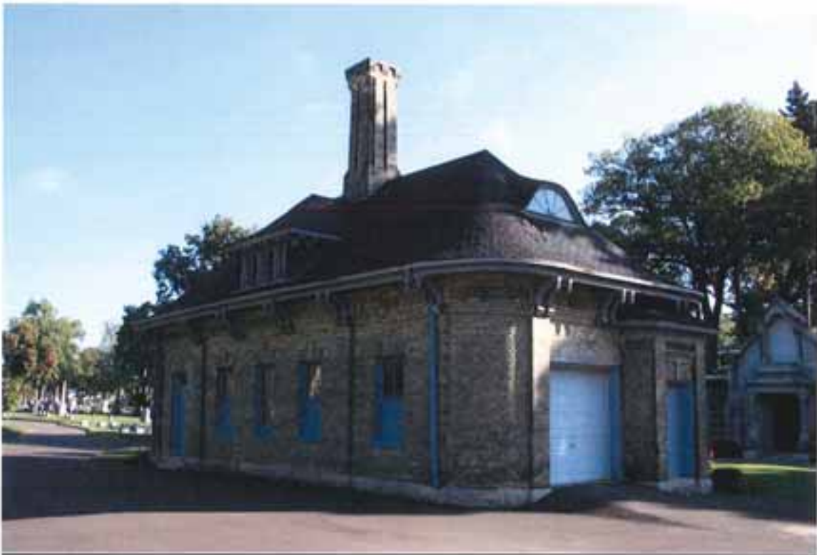
Photograph 11 of 23. Service Building, view facing east.
