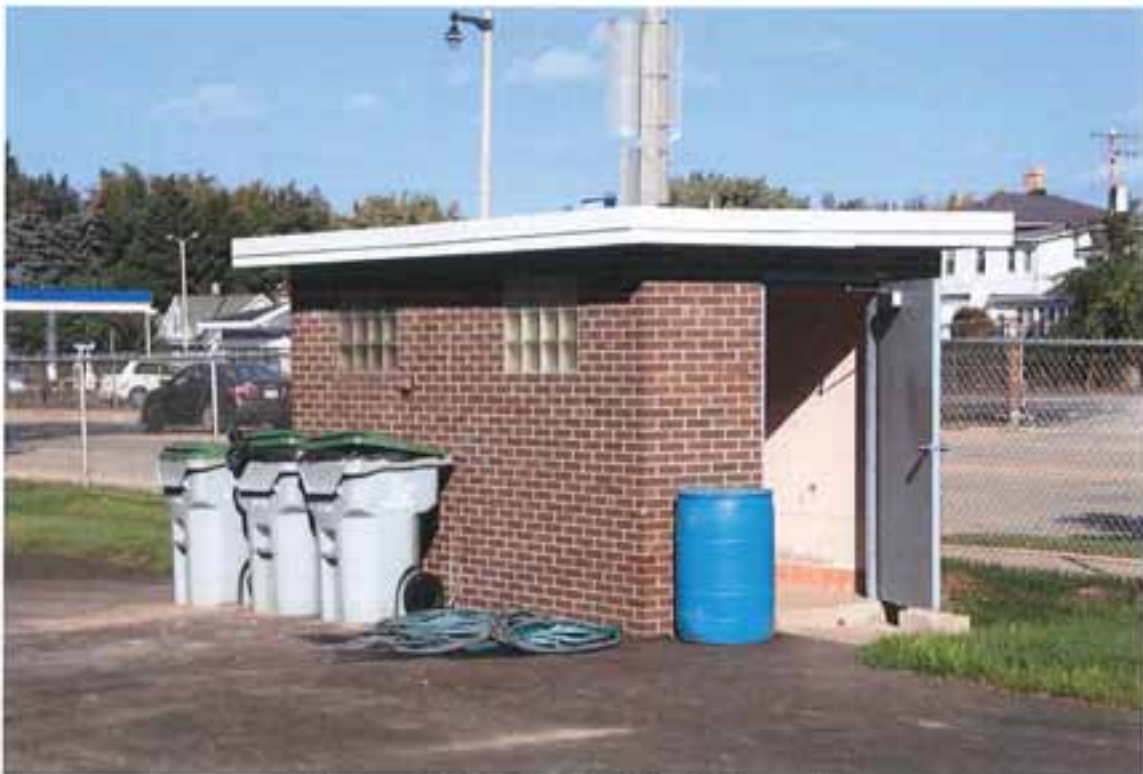
Photograph 23 of 23. Shed, view facing north.
