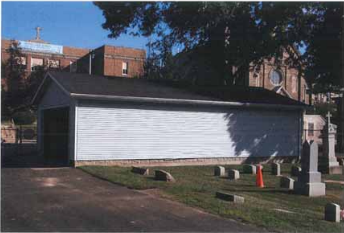
Photograph 22 of 23. Garage, view facing north.
