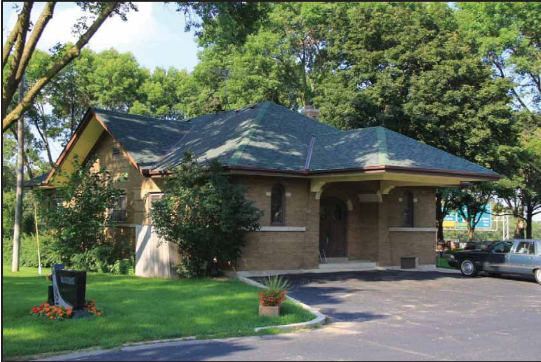
Figure 11 of 12: Spring Hill Cemetery. View to northeast. Former temple, now the caretaker's house.
