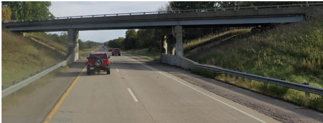
Figure 23. Welch Prairie Road Bridge over EB I-90/94
