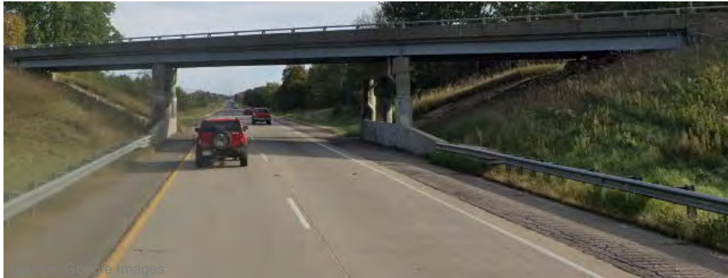
Figure 23. Welch Prairie Road Bridge over EB I-90/94
