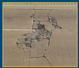
In the fall of 2022, concrete pavement repairs were needed to extend the service life of the pavement. However, adding an overlay is needed to extend the service life and ride quality of the pavement.
