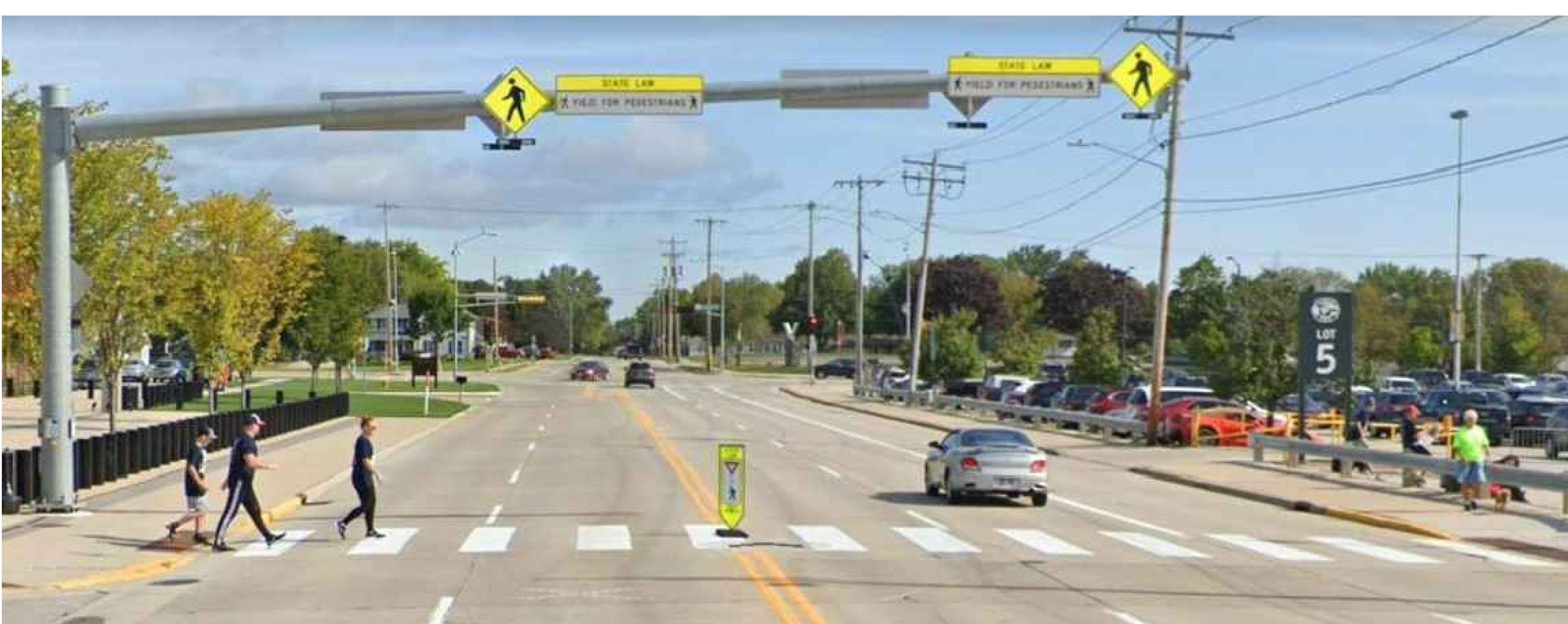
EXAMPLE OF RRFBs USED NEAR LAMBEAU FIELD ON RIDGE ROAD
