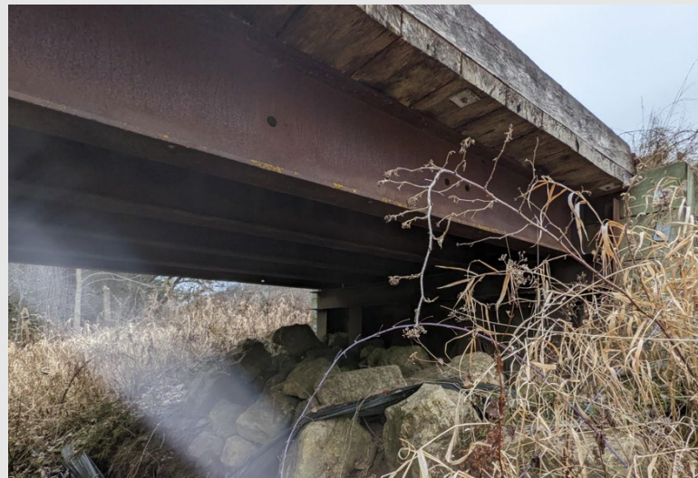
B-52-823, USH 14 bridge over W Branch of Mill Creek
