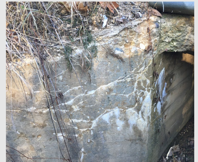
C-52-2025 Box Culvert
