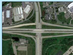
Interchange Example: US 51 & WIS 30
