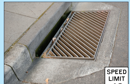
Curb and Gutter
