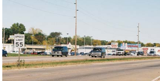
Rural Cross Section: Stoughton Road has a wide cross section typical of rural settings, with limited curb and gutter and a large central swale for drainage and lane separation.
