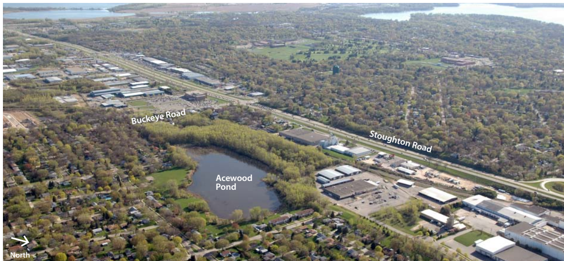
Project Setting: Neighbors and businesses view Stoughton Road as the community’s “main street.” This aerial photograph overlooks the Buckeye Road intersection with South Stoughton Road, just behind Acewood Park and Pond. Lake Monona is on the far right horizon, and Lake Waubesa is on the far left horizon.
