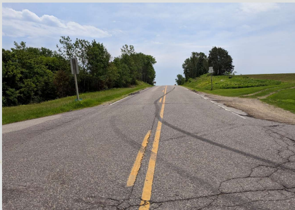
View of blind curve from the County Highway V intersection
