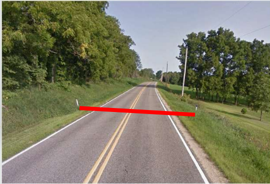
Culvert pipe 1.49 miles north of County Highway J
