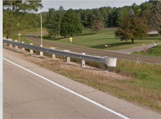
Existing end of guardrail on WIS 113
