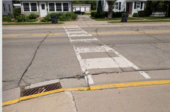
Crosswalk at the First Street intersection crossing WIS 113
