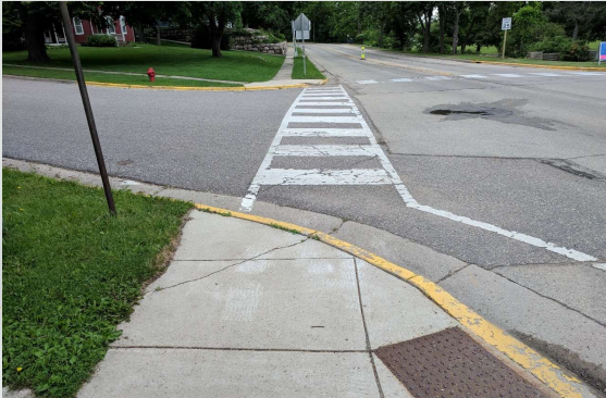
Crosswalk at the Chestnut Street intersection crossing Chestnut Street
