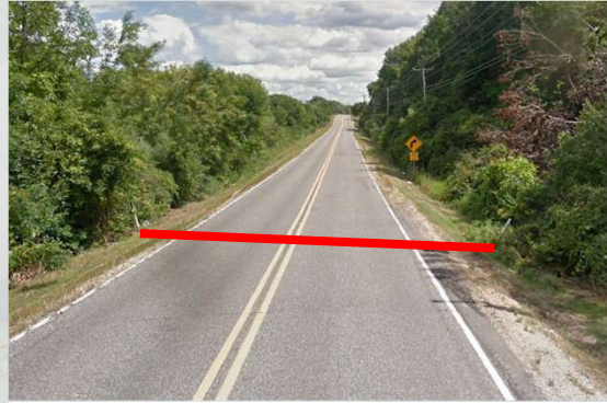
Culvert pipe 0.75 miles north of Old Sauk Road
