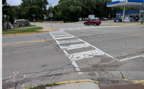
Crosswalk at the Chestnut Street and Fair Street intersection crossing WIS 113
