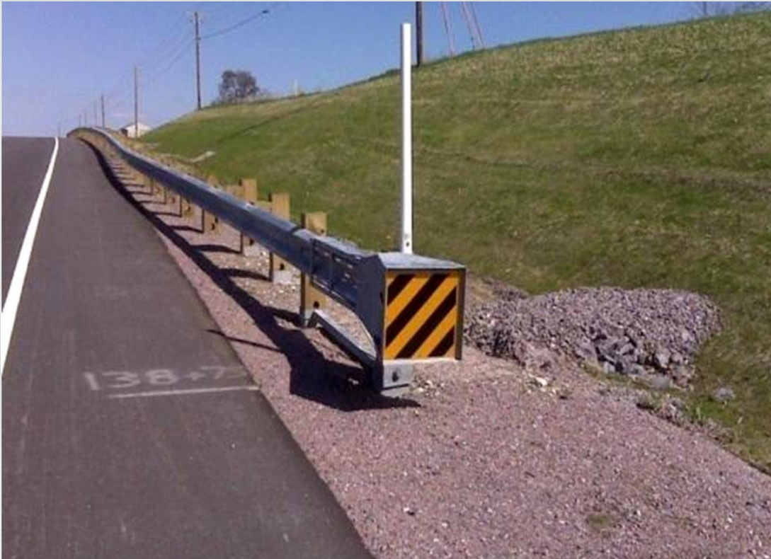
Energy Absorbing Terminal (EAT)
