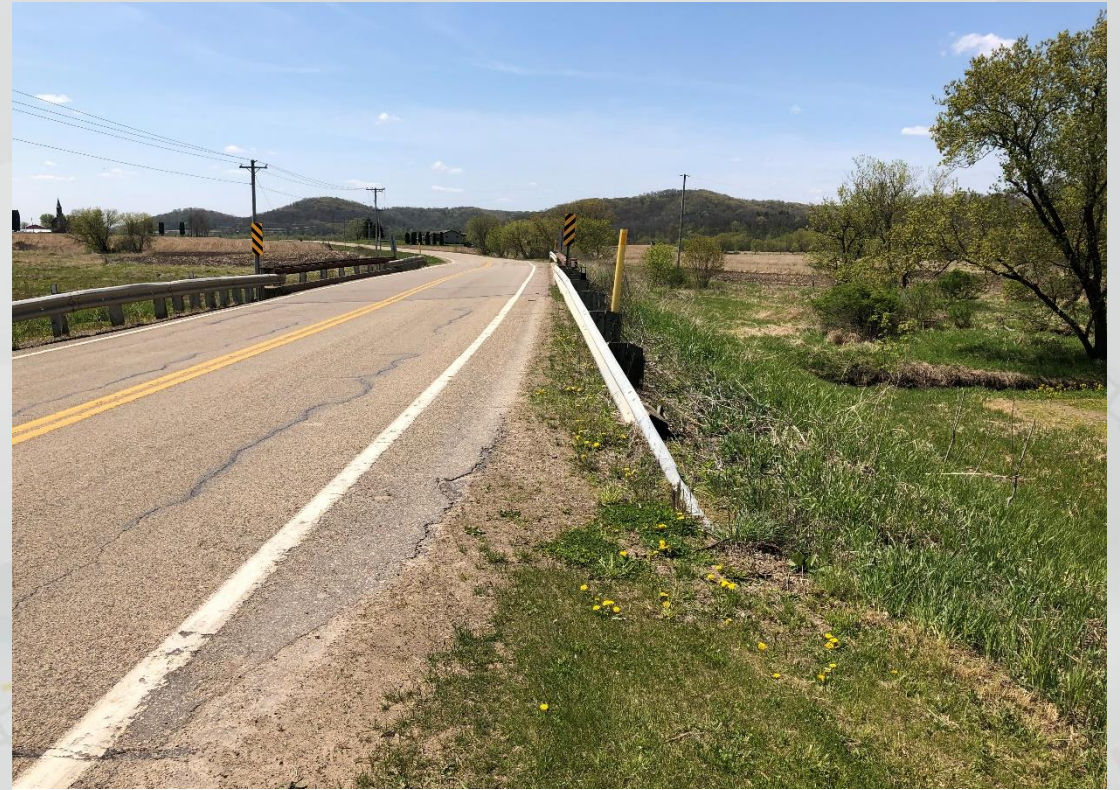
Existing end of guardrail on WIS 130
