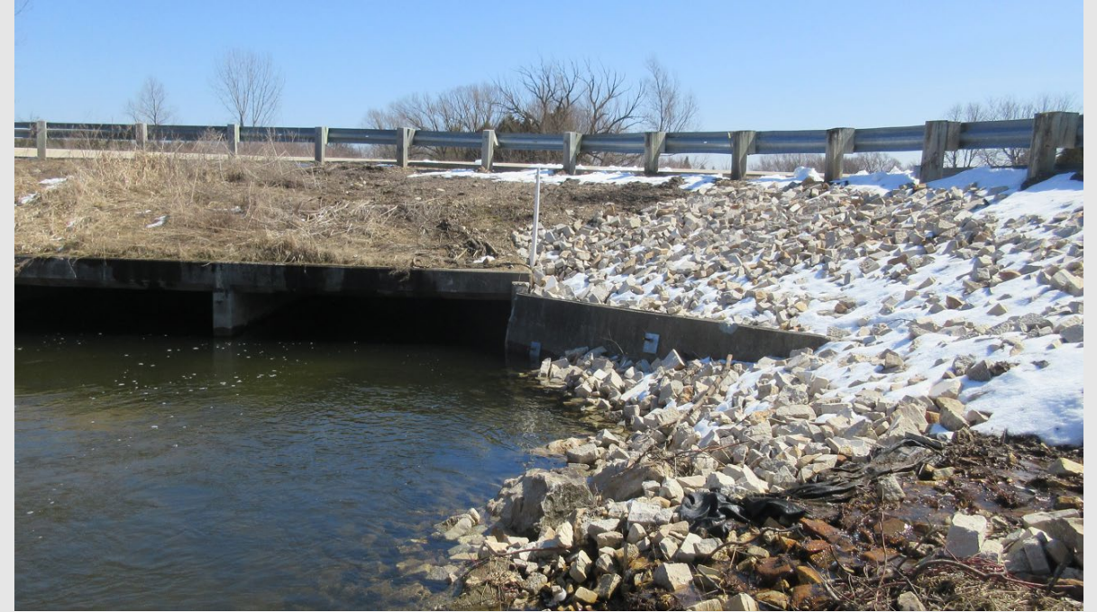
At Zion Church Rd
