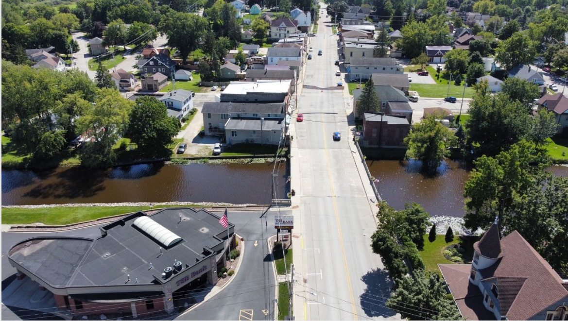
Bridge over Rock River
