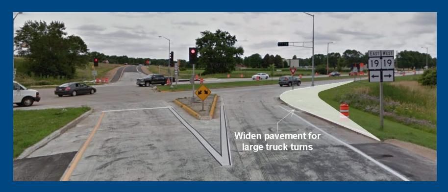
By providing wider pavement, large trucks will have more room to turn right onto westbound WIS 19 without driving over the curb resulting in less damage to trucks, the splitter island, traffic signs, and the signal/light pole.
