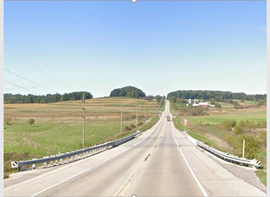
Substandard Guardrail Terminal Ends / Insufficient Guardrail Height
