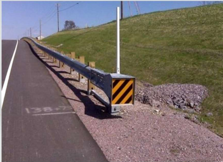
Energy Absorbing Terminal (EAT)
