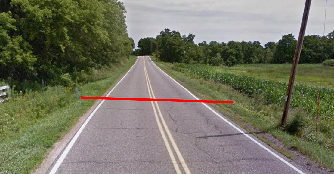
Culvert Pipe 0.08 miles north of Richland-Sauk Co Line
