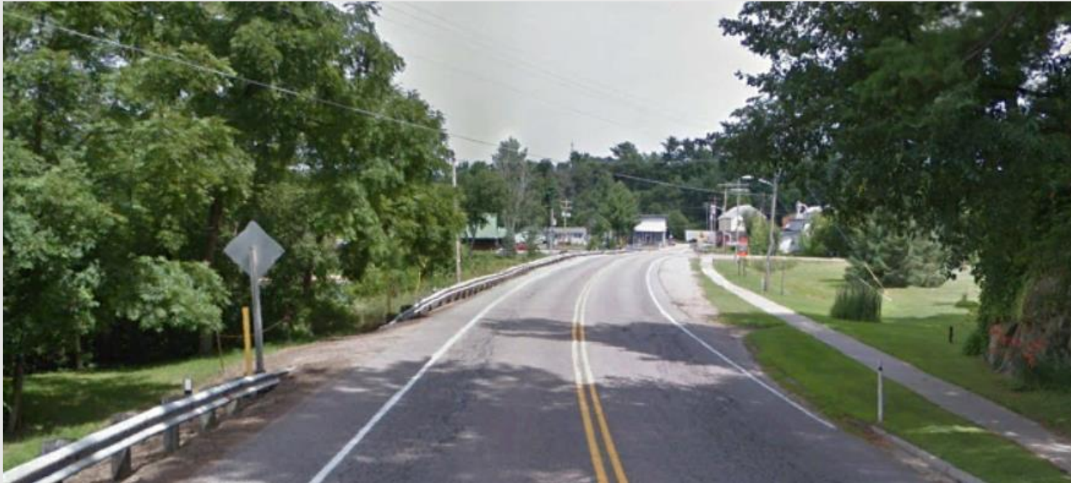
La Valle Mill Pond – 375' Pavement Reconstruct
