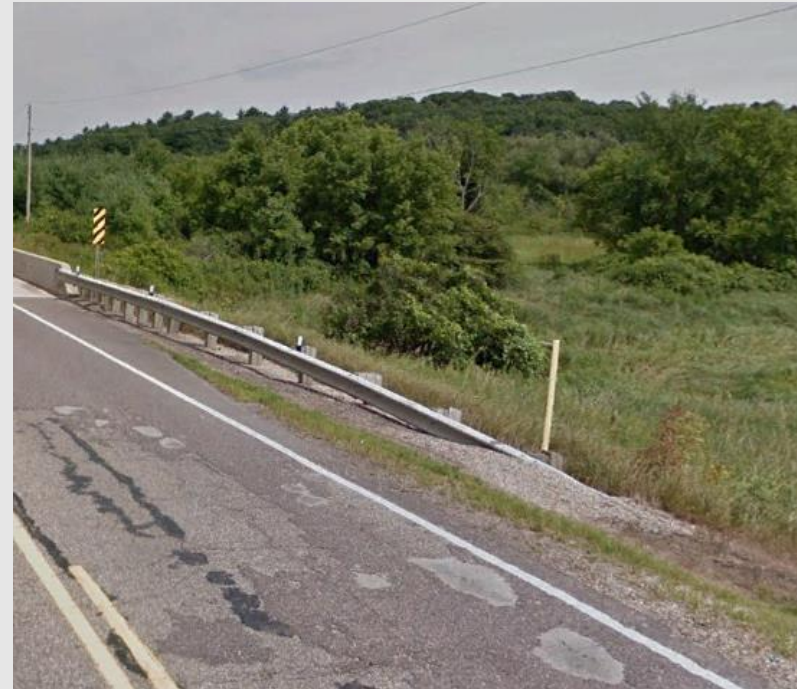
Existing end of guardrail on WIS 58
