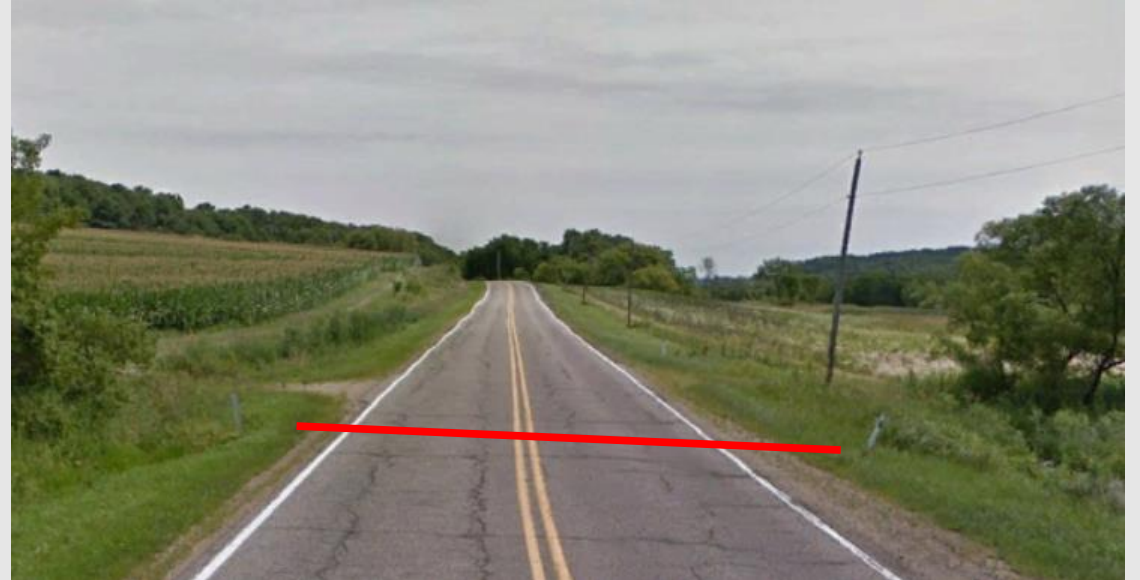
Culvert Pipe 0.35 miles north of Richland-Sauk Co Line
