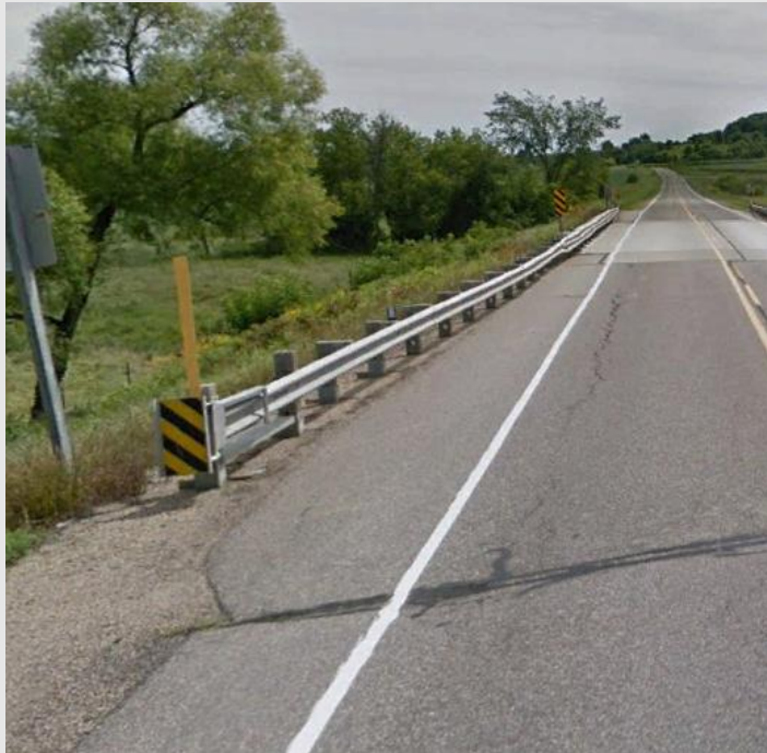
Energy Absorbing Terminal (EAT)
