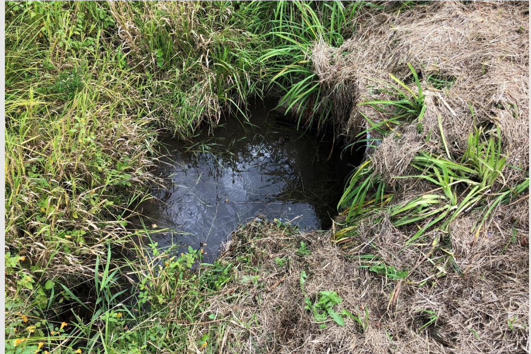
36-inch culvert pipe 0.35 miles north of Richland-Sauk Co Line
