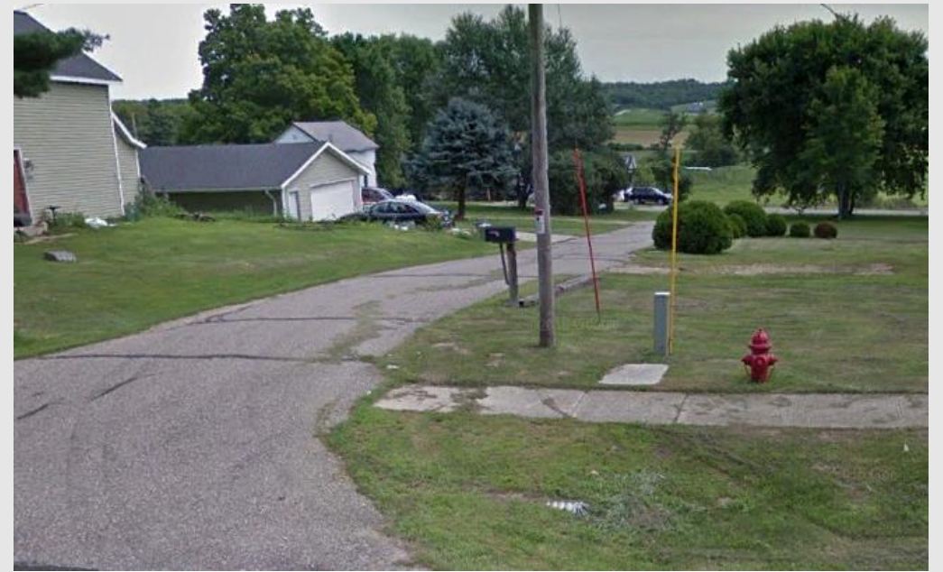
Crossing at 4 th Street in Ironton
