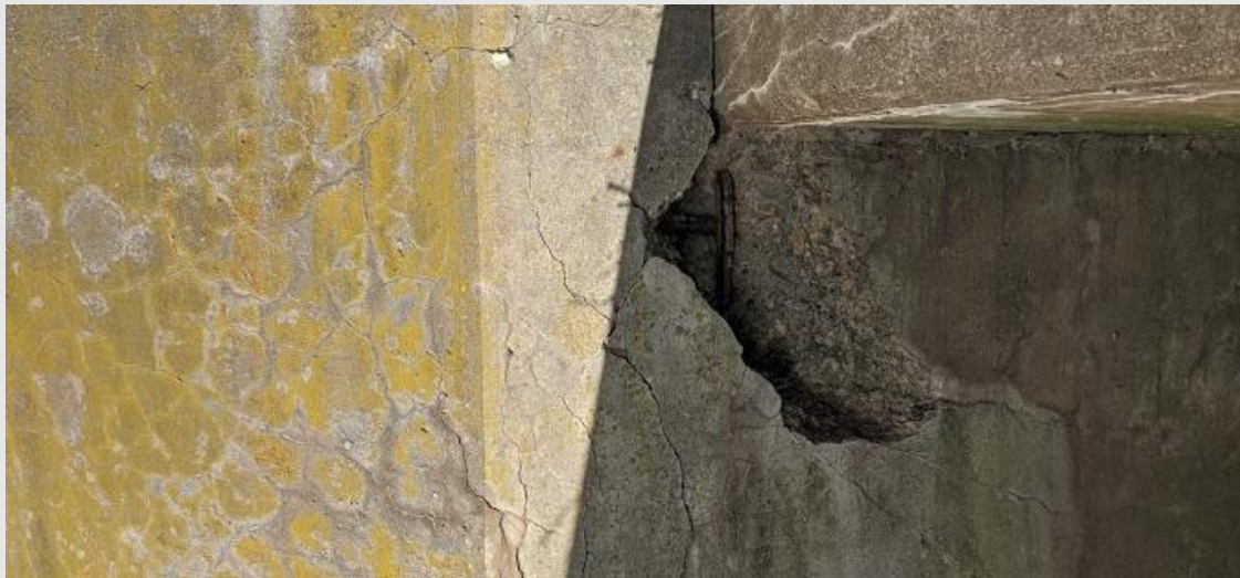
Box Culvert C-11-2027
