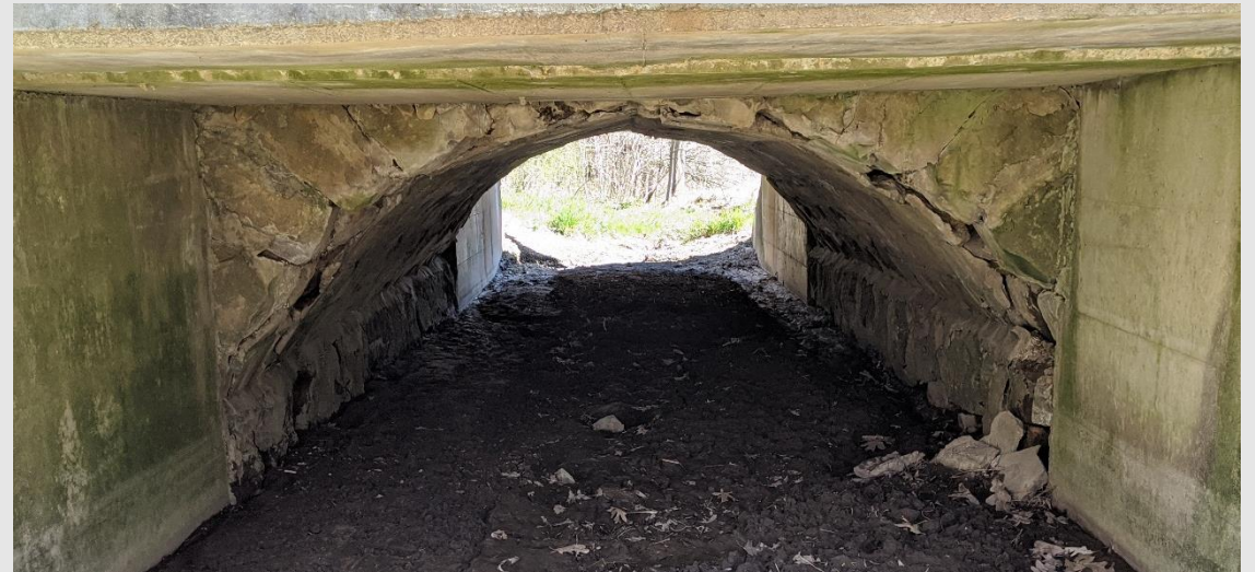
Box Culvert C-11-3005
