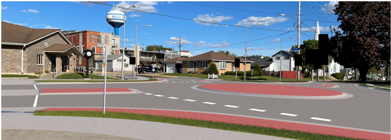
Rendering of the proposed compact roundabout at WIS 80/WIS 11 in Hazel Green – looking southeast
