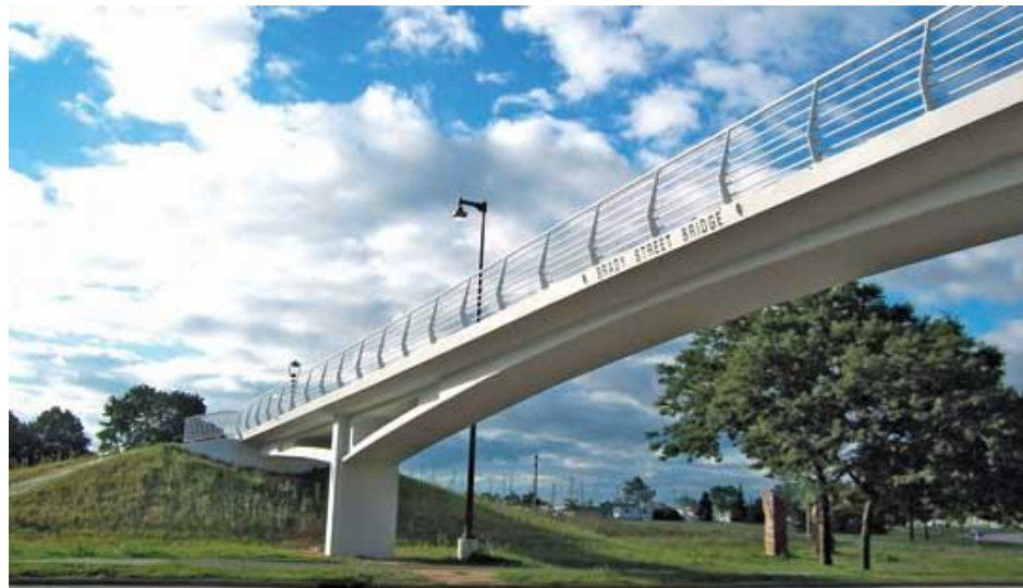
Figure 1: Brady Street Pedestrian Bridge
