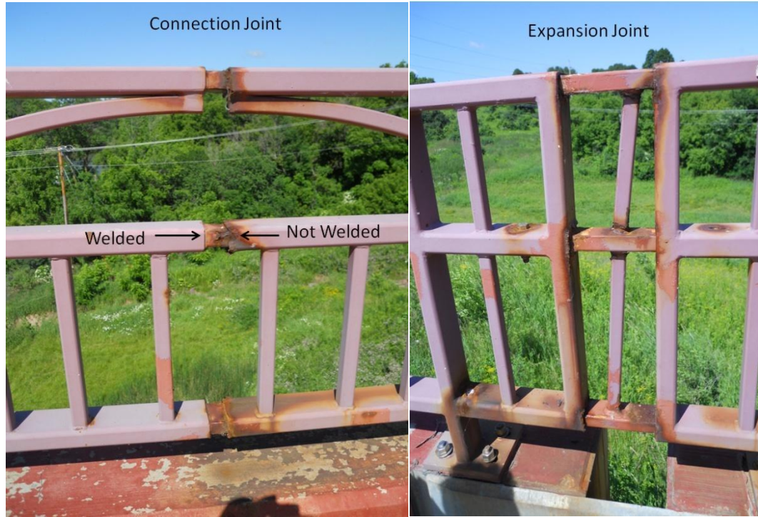
Figure 4: Baraboo Bridge Railing Connection/Expansion Joint
