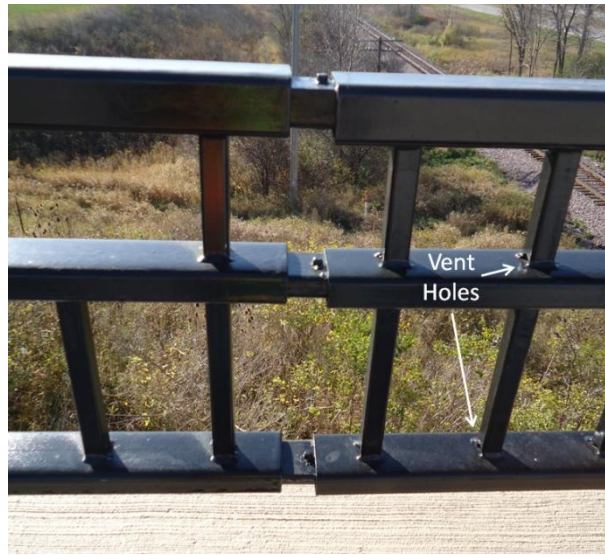
Figure 13: Highland Ave and I-43 Bridge Railing Vent Holes
