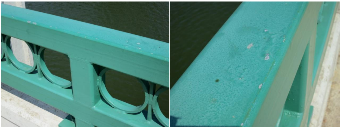
Figure 16: Beloit Bridge Railing Galvanized Railing
