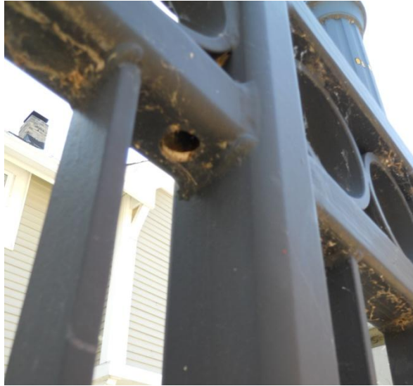
Figure 11: Jefferson Bridge Railing Galvanization Holes
