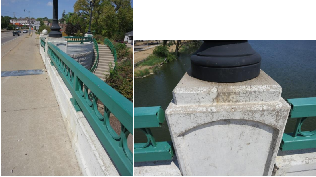
Figure 17: Beloit Bridge Railing Connections
