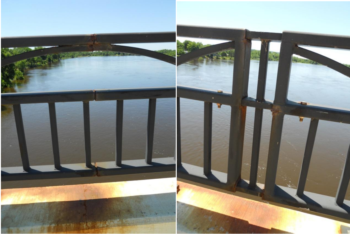
Figure 6: Sauk City Bridge Railing Connections
