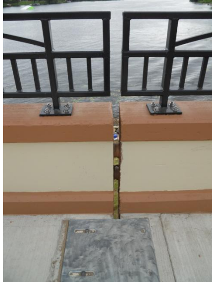
Figure 12: Tomahawk Bridge Railing Expansion Joint
