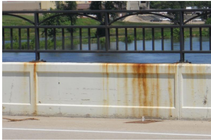
Figure 2: Sauk City, WI Bridge
