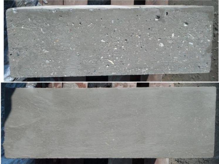
Figure 0-3: Concrete specimen before and after sack rubbing surface treatment.
