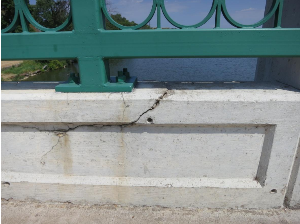
Figure 0-6: Voids left in concrete surface to accommodate form ties.
