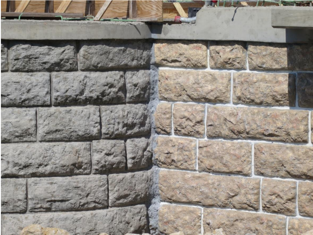
Figure 0-1: Prepared and coated form lined concrete surfaces.
