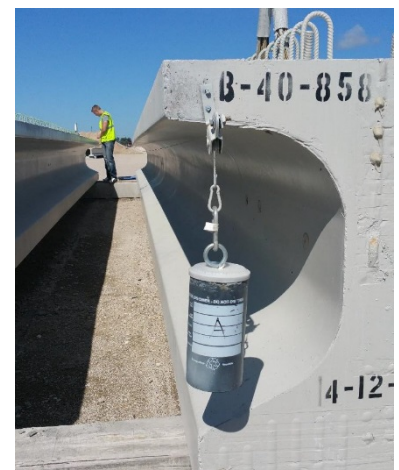
Camber was measured early in the morning to mitigate thermal effects.
