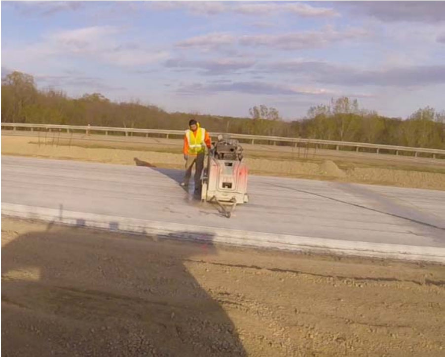
Figure 2.2.6: Transverse Saw Cutting with the Husqvarna 6600D Conventional Saw
