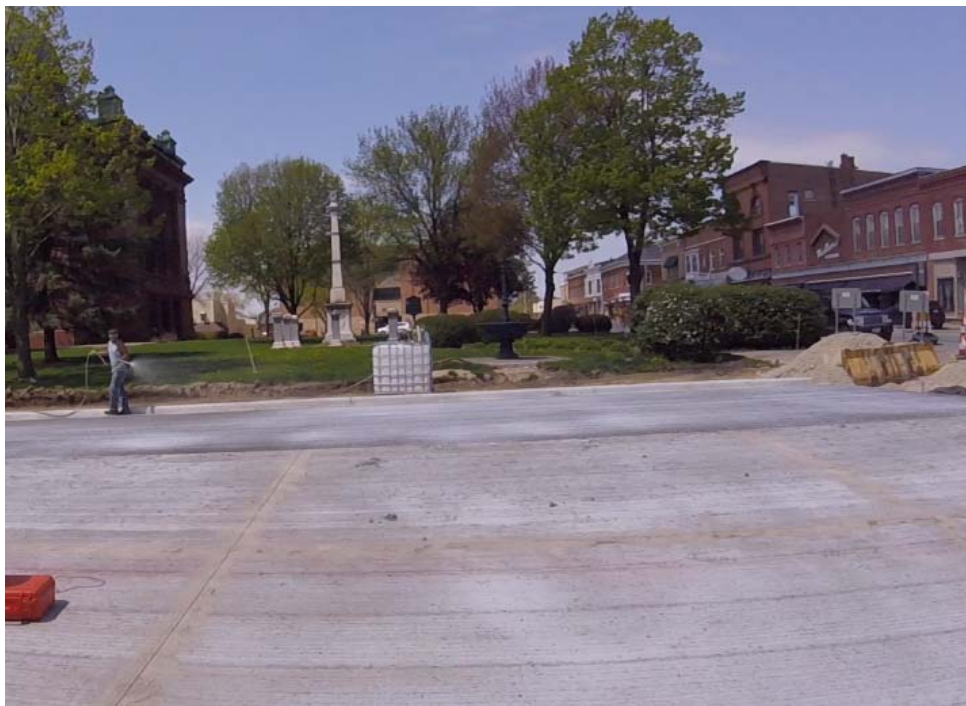
Figure 2.3.4: Hand Spray Application of Curing Compound
