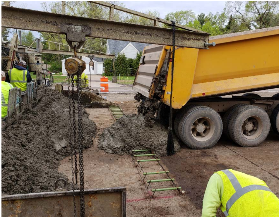
Figure 2.4.2: Concrete Placement Over Dowel Baskets
