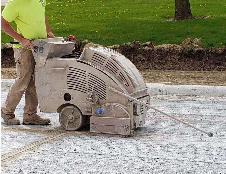
Figure 2.3.6: Longitudinal Joint Saw Cutting
