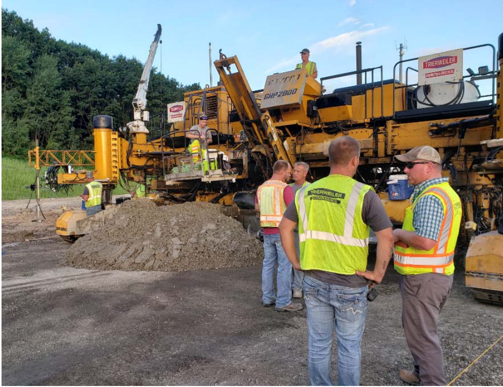
Figure 2.5.1: First Load Placement at 5:57 AM
