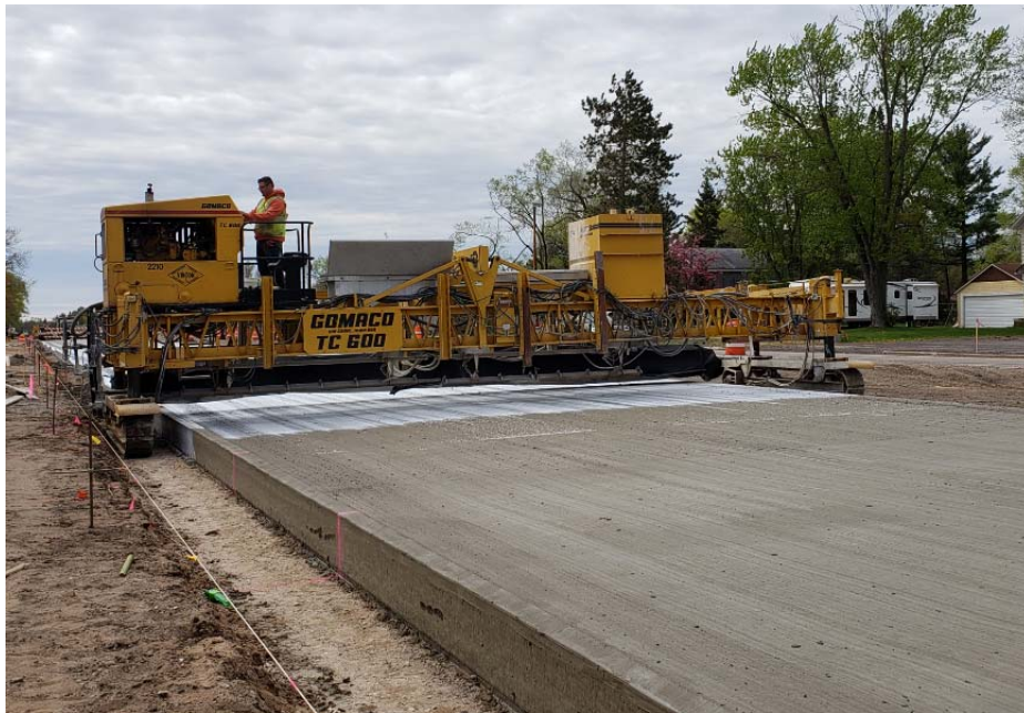
Figure 2.4.4: Application of Curing Compound
