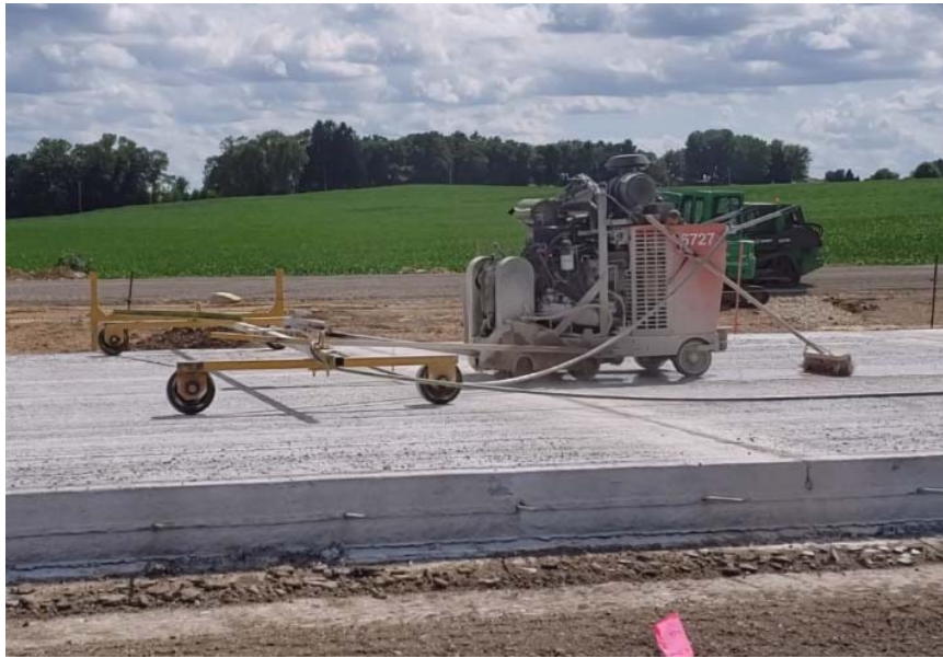
Figure 2.5.7: Longitudinal Joint Saw Cutting with the Guided FS 8500D
