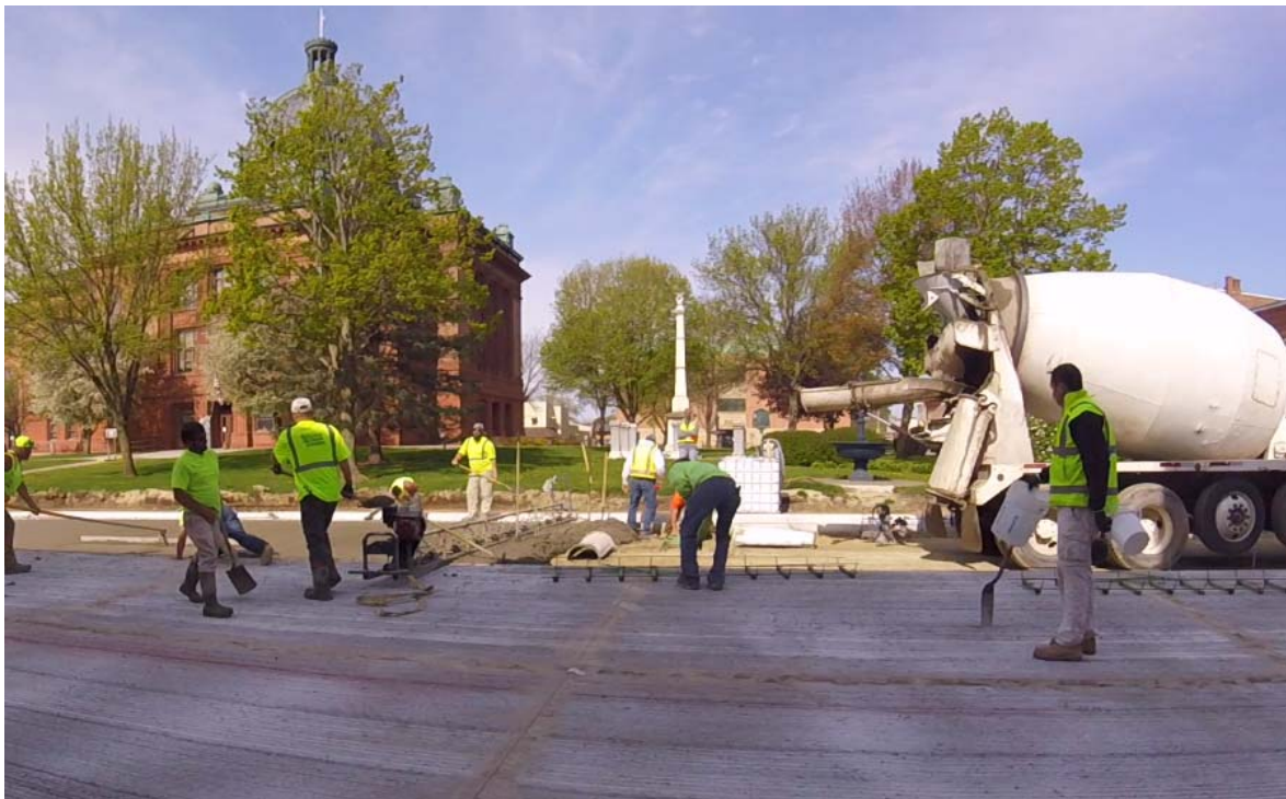
Figure 2.3.2: Concrete Placement Near Monitoring Location
