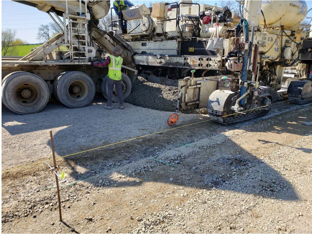
Figure 2.2.1: First Load of Concrete on USH 151
