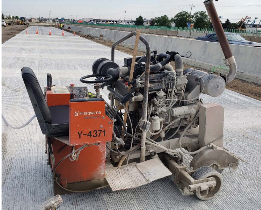
Figure 2.6.5: Transverse Joint Sawing with the Husqvarna RS 8500D
