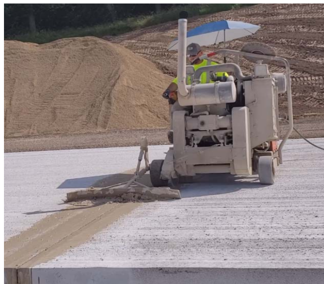
Figure 2.5.6: Slurry Push-Off with the Rubber Plow
