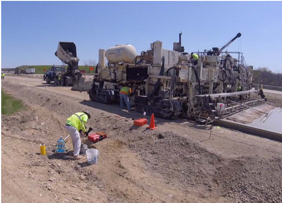
Figure 2.2.4: Paving and Testing Operations at the Monitoring Joint
