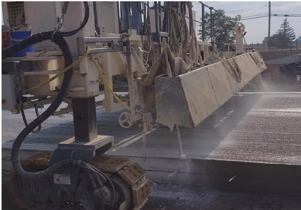
Figure 2.6.4: Application of Curing Compound
