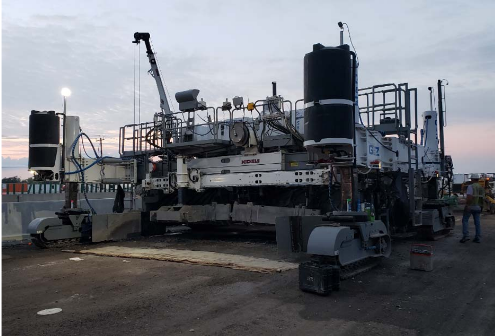
Figure 2.6.1: Paver Ready for First Load at 5:20 AM
