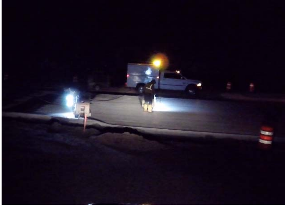
Figure 2.4.7: Tandem Transverse Joint Saw Cutting
