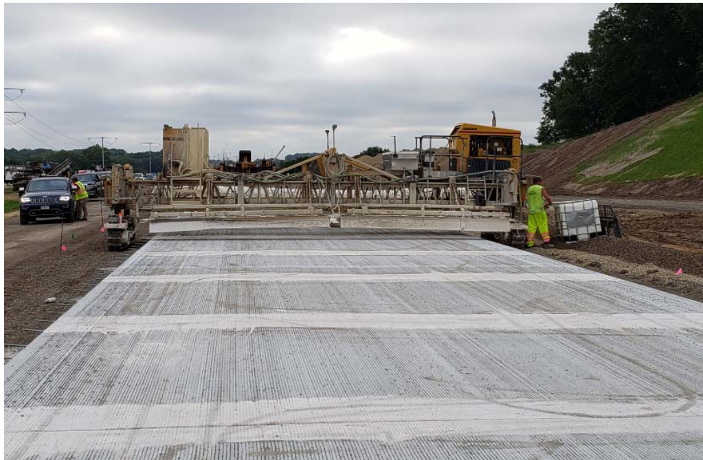
Figure 2.5.4: Application of Curing Compound
