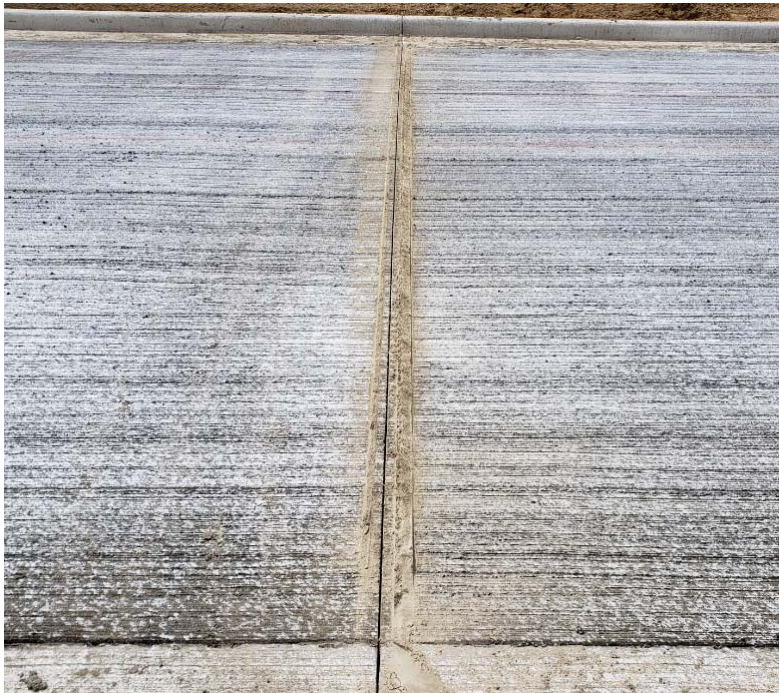
Figure 2.3.7: Finished Transverse Joint Saw Cut
