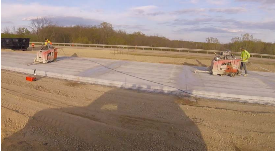
Figure 2.2.7: Transverse and Longitudinal Saw Cutting
