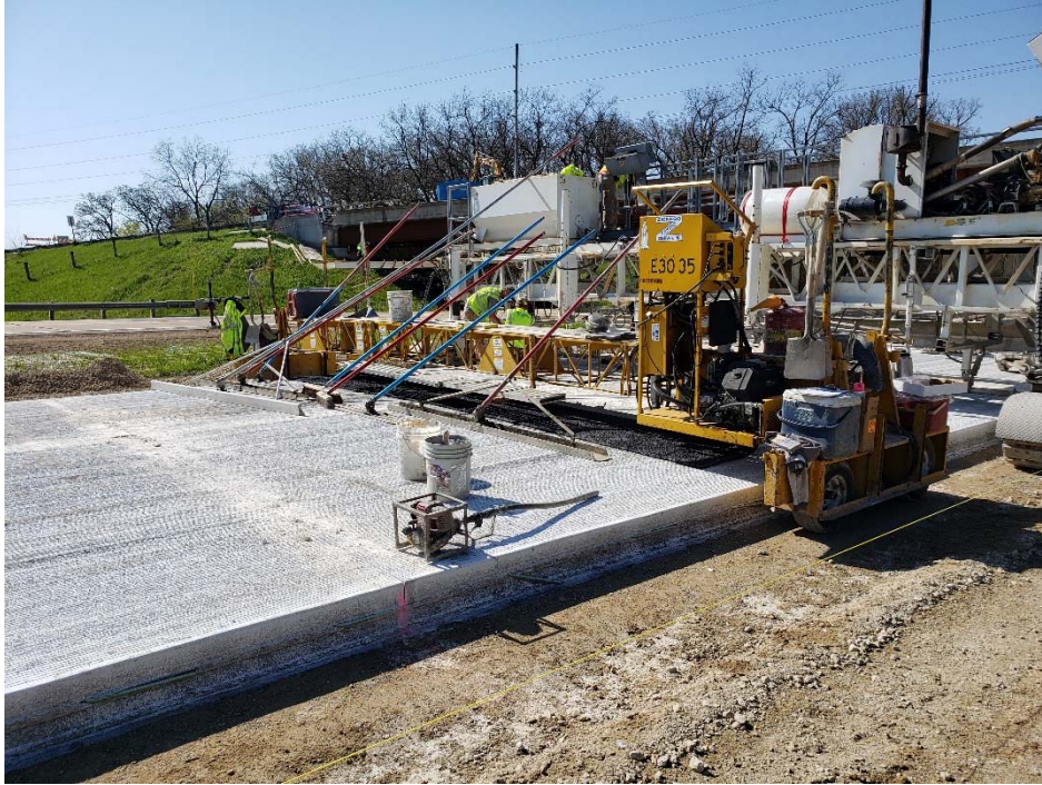
Figure 2.2.3: Pavement Texturing and Curing Compound Equipment
