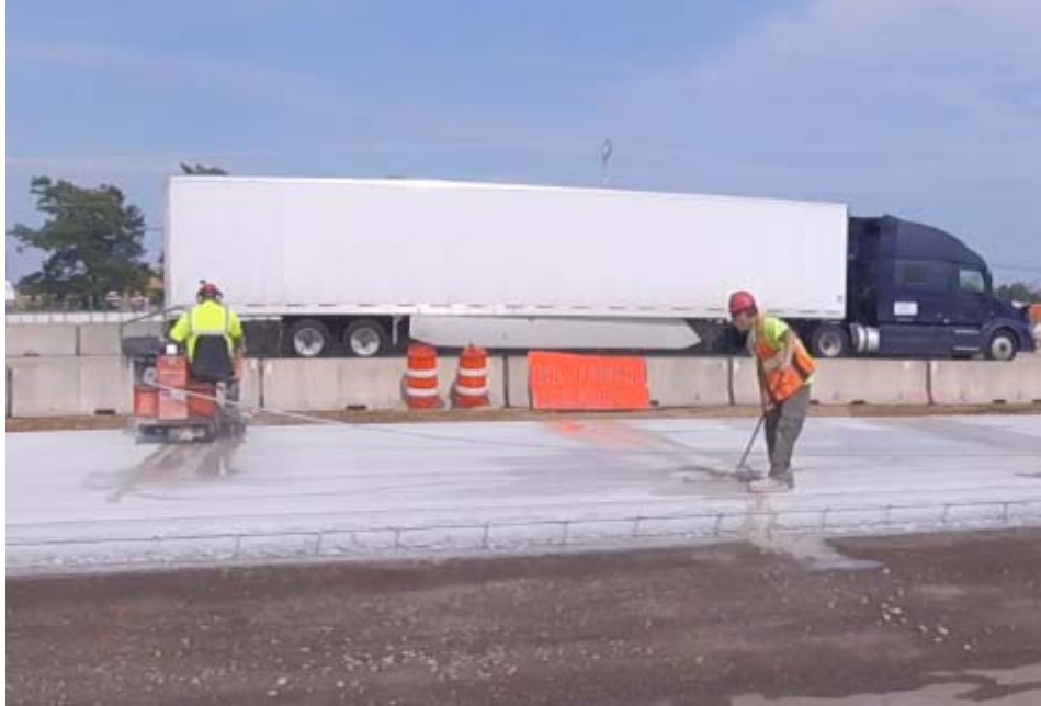
Figure 2.6.7: Slurry Push-Off with the Rubber Plow
