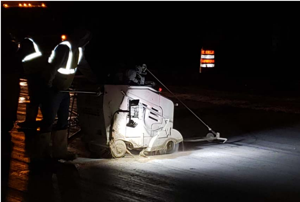
Figure 2.4.6: Transverse Joint Saw Cutting
