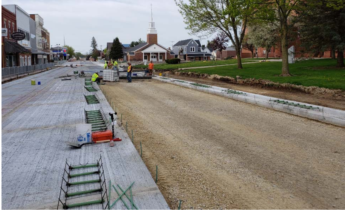
Figure 2.3.1: USH 61 (Madison St.) Paving Site Prior to First Load of Concrete
