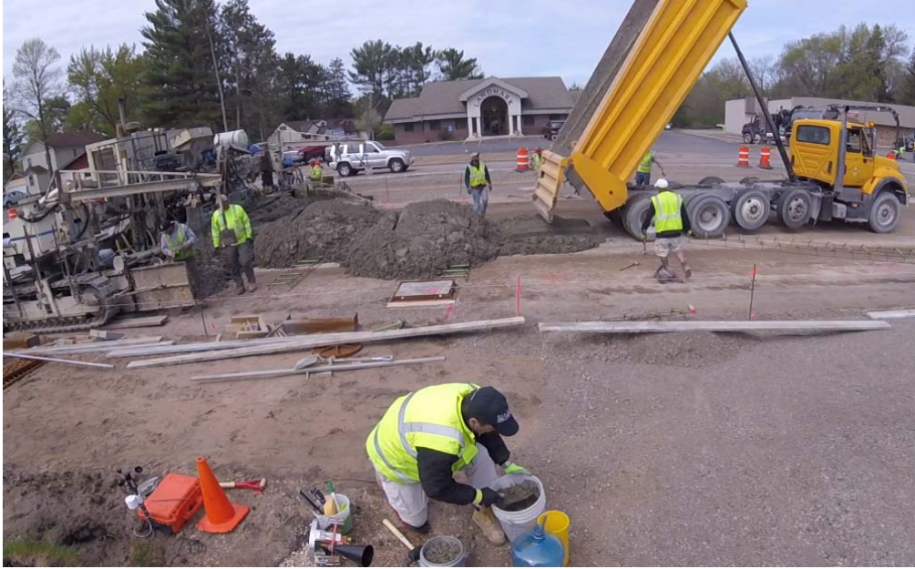
Figure 2.4.1: Concrete Placement Near Monitoring Location
