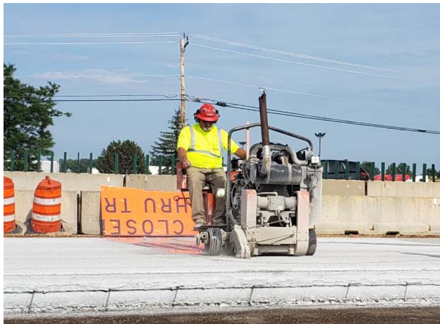
Figure 2.6.6: Transverse Joint Sawing with the Husqvarna RS 8500D
