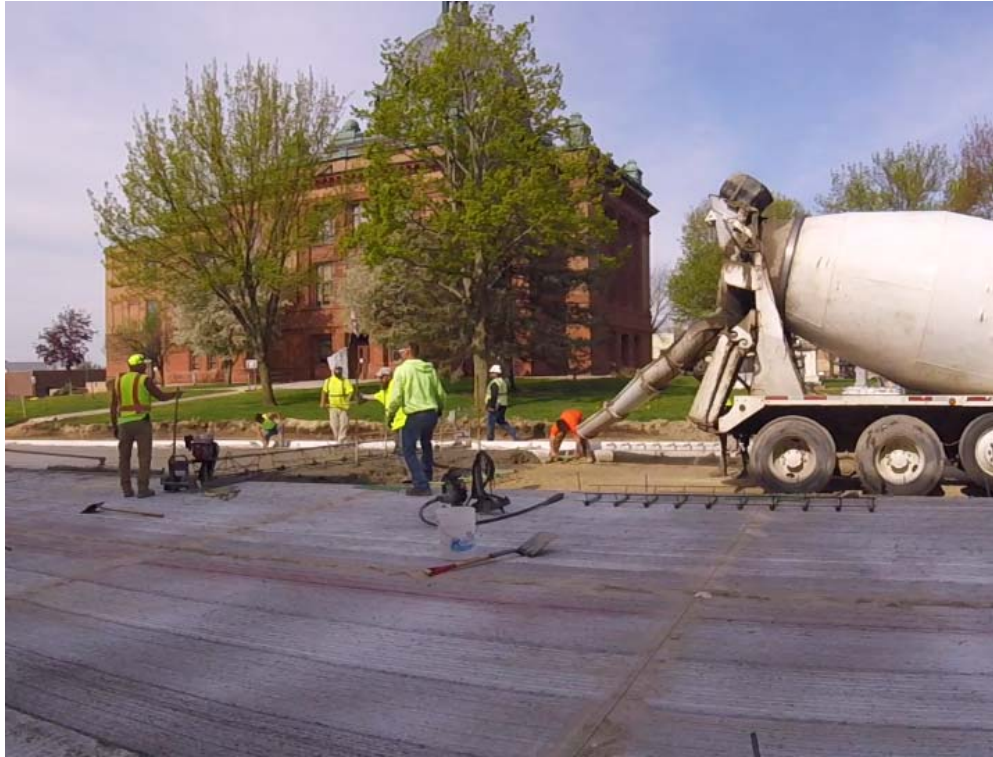
Figure 2.3.3: Dowel Basket Placement and Vibrating Screenshot
