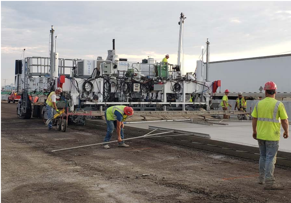
Figure 2.6.2: Stringless Paving Operations
