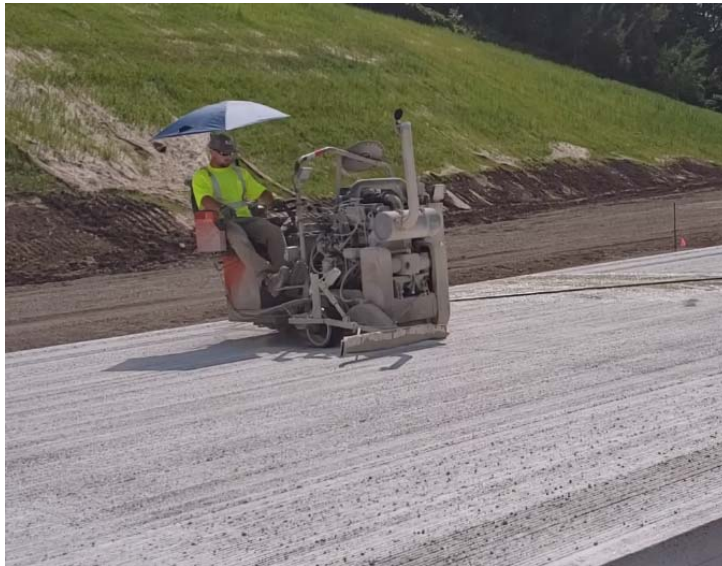
Figure 2.5.5: Transverse Joint Sawing with the Husqvarna RS 8500D
