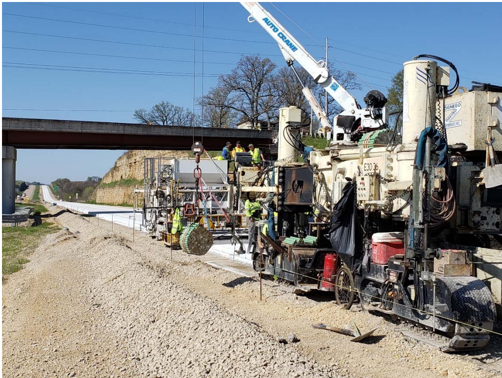
Figure 2.2.2: Dowel Bar Handling Prior to Insertion
