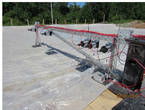
Instrumentation to monitor deflection set over curing concrete.
