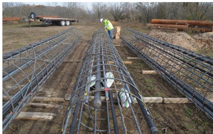
Reinforcing cages prepped with sensors and sandbags
