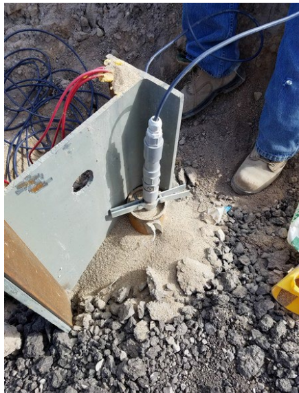
A Shaped Array Accelerometer secured at ground level.
