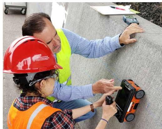
Ground penetrating radar is used to locate rebar within barriers.
