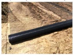
Geogrid material and aperture shapes vary by manufacturer, and there are multiple test methods for determining strength. WisDOT currently uses ASTM D4595, which was originally developed for geotextiles, a different type of geosynthetic. ASTM D6637 Method B has gained popularity, as agencies and
