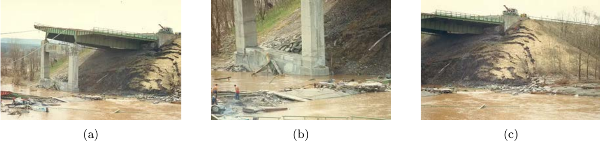
Figure 1: Photos from a Utica resident document the aftermath of the collapse of the New York State Thruway bridge over the Schoharie Creek in 1987 [29]
