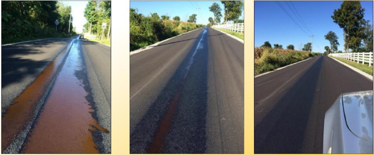
Figure 16. Rapid Penetrating Emulsion used as a longitudinal joint preventative treatment immediately following application (left), after penetrating joint (center), and dried (right). (19).
