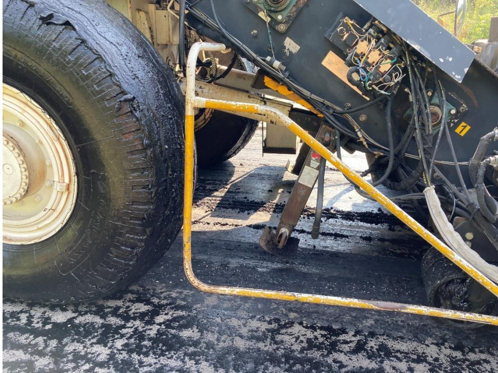
Figure 15. Pickup of tack coat residue on paving tires and removal from substrate. Author photo.
