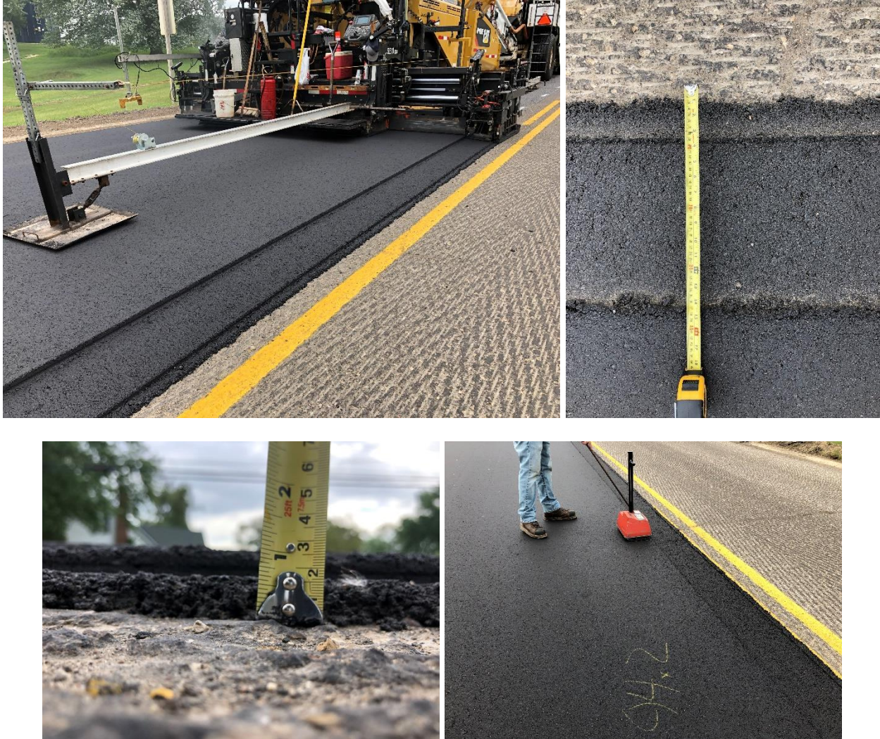
Figure 2. Wisconsin Notched-Wedge Joint construction practice including unconfined joint density measurement by nuclear method.
