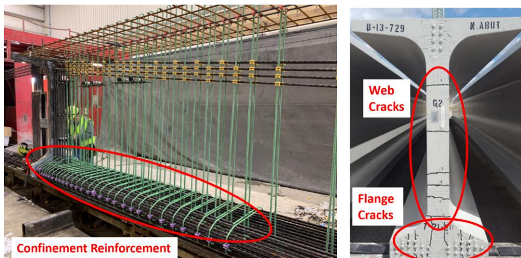
Figure 36 - Girder reinforcement prior to casting concrete (left) and representative end cracking (right).
