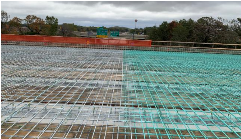
Figure 35 - Photo of the deck before casting concrete (looking east).
