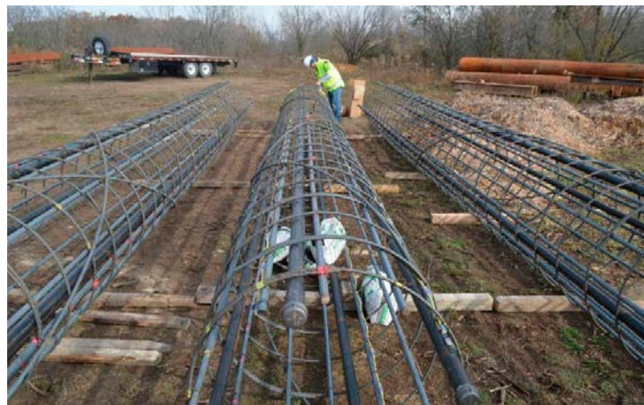
Reinforcing cages prepped with sensors and sandbags
