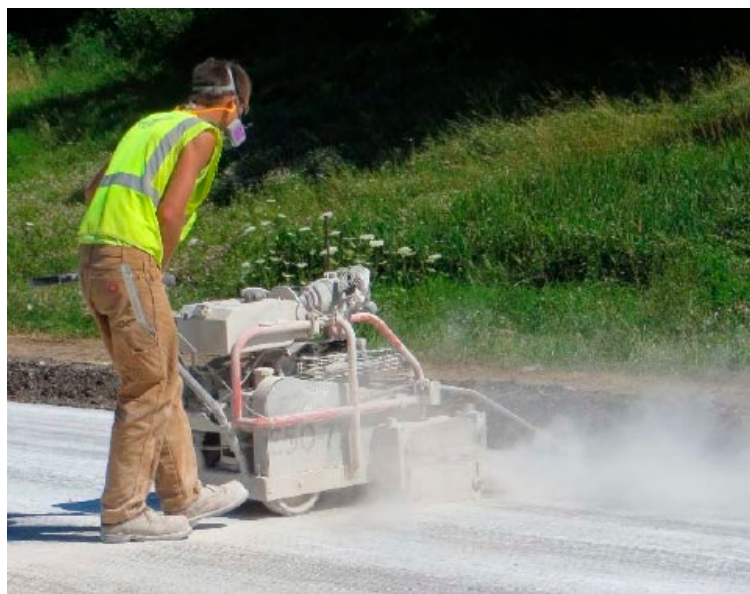
Performing an early-entry saw cut
