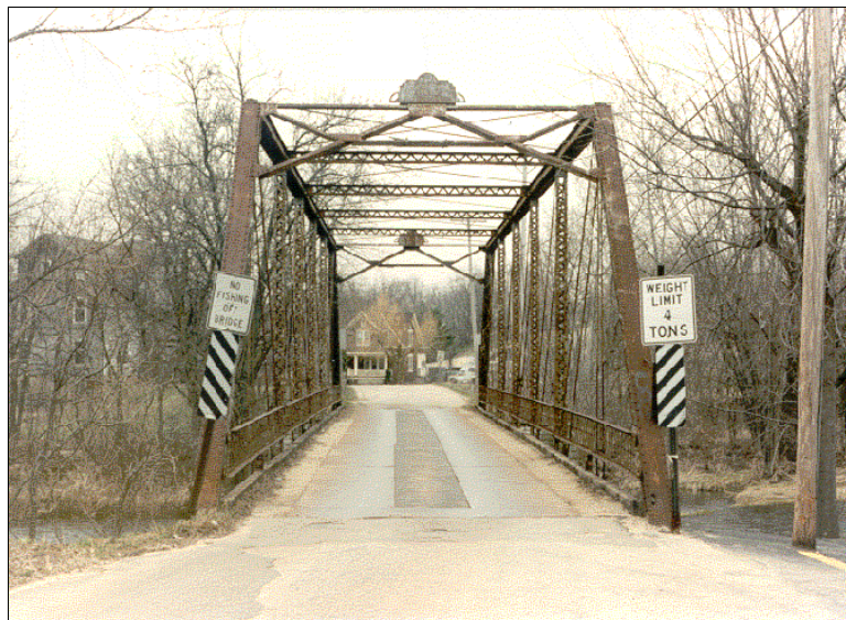
Figure 1.3.13.1-2: Load Posted Truss Bridge.
