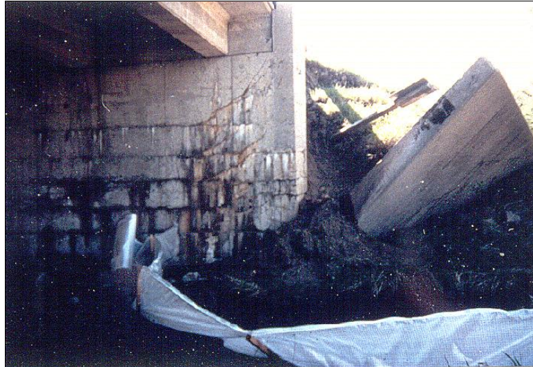
Figure 1.3.12.1-2: Failed Wingwall.
