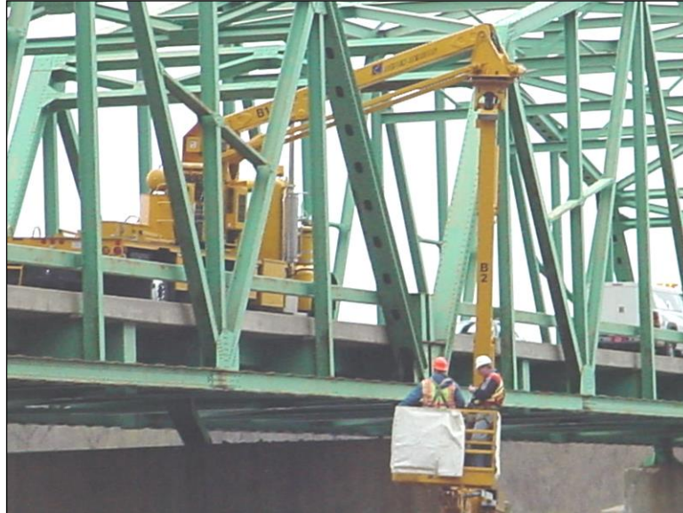
Figure 1.3.5.1-1: Inspectors Performing a NSTM Inspection
