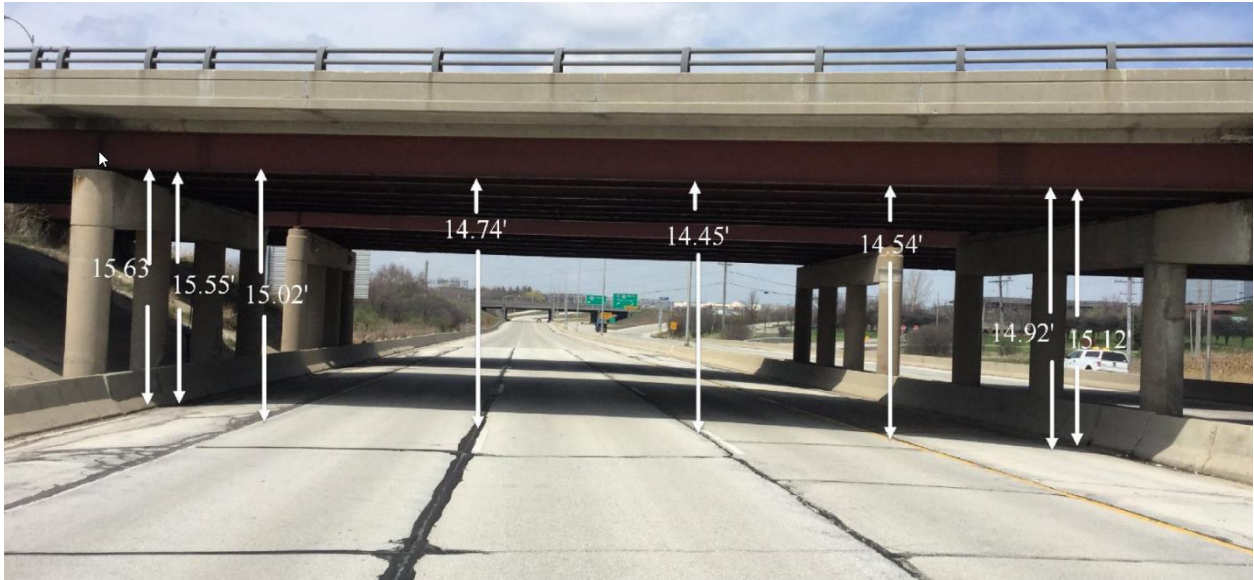
Figure 1.3.15.1-1: Vertical Clearance Photo
