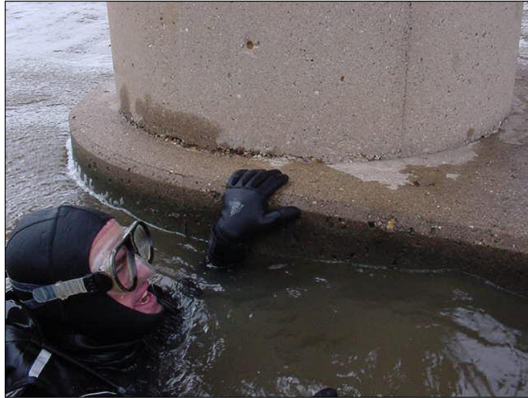
Figure 1.3.8.2-2: Inspector Conducting a Level I Inspection Effort.
