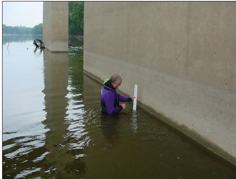
Figure 1.3.9-1: Inspector Conducting a Wading Inspection.
