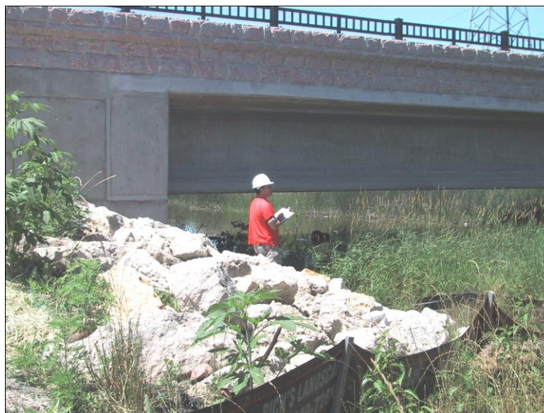
Figure 1.3.2.1-1: Inspector Performing an Initial Inspection.
