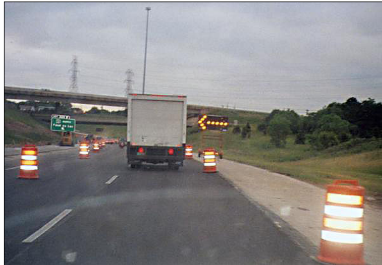
Figure 1.4.8.3-2: Directional Arrow Board and Channelizing Barrels.
