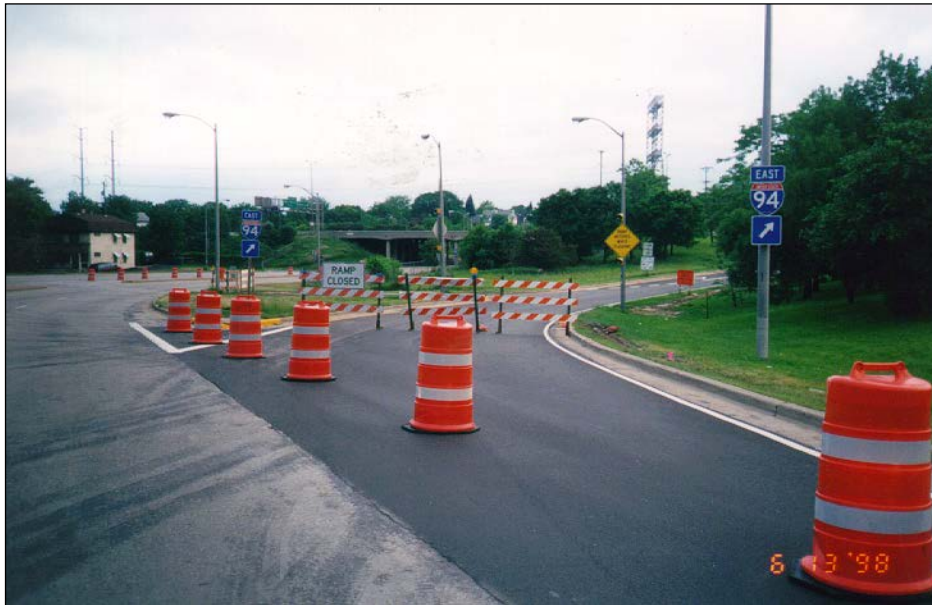
Figure 1.4.8.1-1: Barrels Channel Traffic Away From Work Zone.
