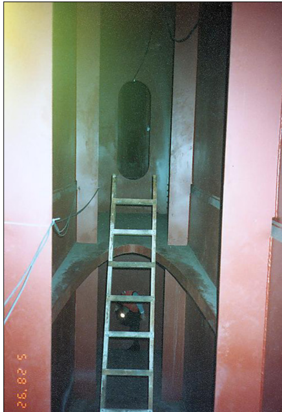
Figure 1.4.3.2-2: A View Inside of a Steel Box Girder.
