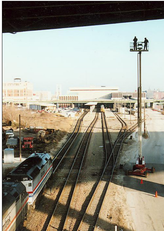
Figure 1.4.3.2-1: Inspectors Working Next to a Live Railway.
