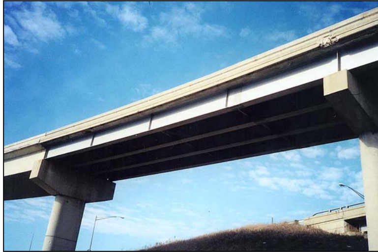
Figure 2.1.5.2-1: Steel Multiple Girder Bridge.
