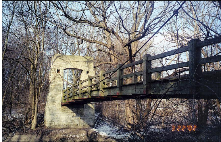
Figure 2.1.5.7-1: Pedestrian Suspension Bridge.
