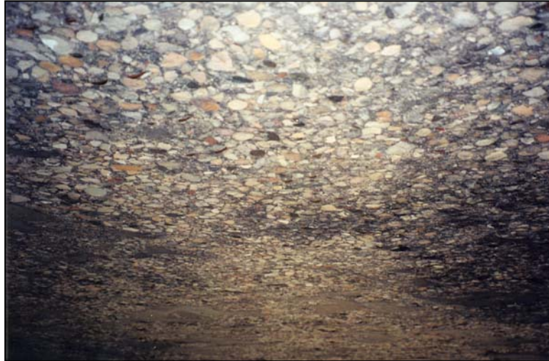
Figure 2.1.4.1-9: Scaling on the Underside of a Concrete Box Girder Due to Fire.
