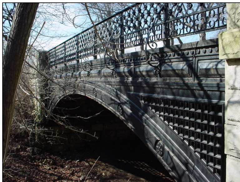
Figure 2.1.4.4-3: Cast Iron Arch.
