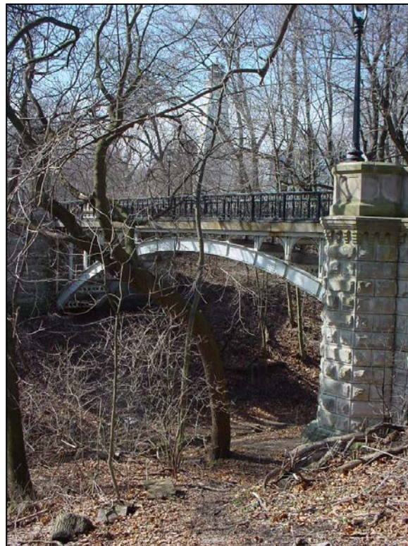
Figure 2.1.5.4-2: Steel Open Spandrel Arch.
