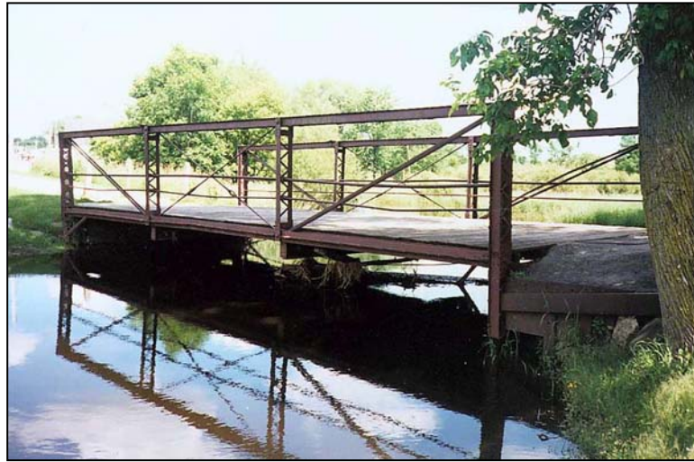
Figure 2.1.5.3-3: Pratt Truss Bridge.
