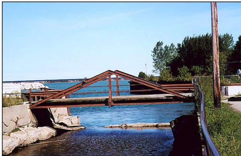
Figure 2.1.5.3-2: King Post Truss Bridge.
