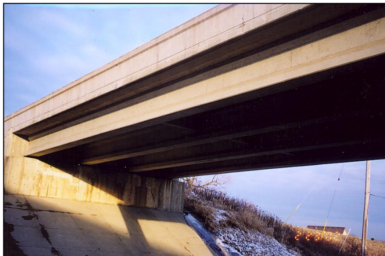
Figure 2.1.5.2-2: Prestressed Concrete Multiple Girder Bridge.
