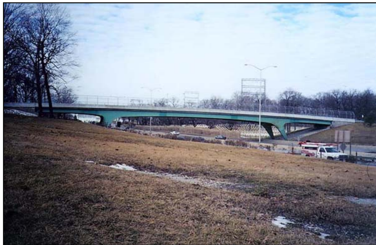
Figure 2.1.5.5-1: Steel Rigid Frame.
