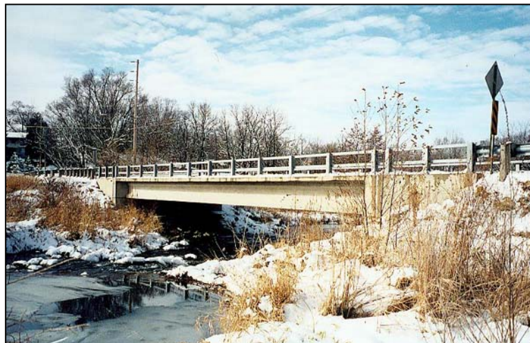
Figure 2.1.2.2-1: Simply Supported Span – Prestressed Concrete Girders.
