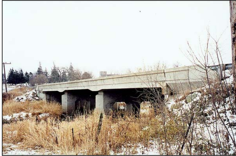
Figure 2.1.5.1-2: Three-Span Concrete Slab with Haunches.
