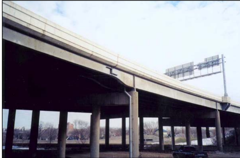
Figure 2.1.2.4-1: Steel Cantilever Span.
