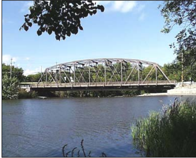
Figure 2.1.5.3-1: Parker Truss Bridge.
