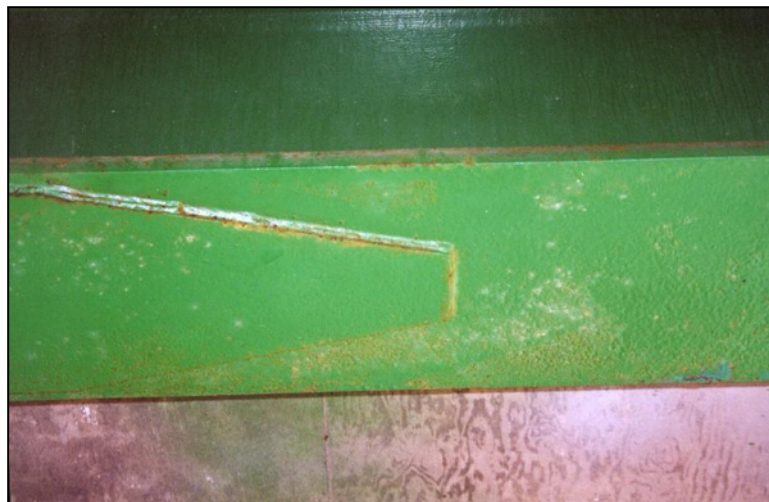
Figure 2.1.4.2-2: Transverse Weld at a Cover Plate End.
