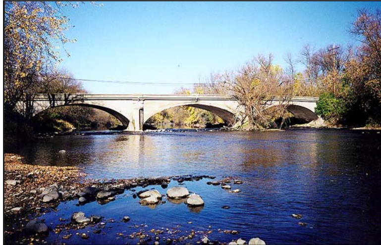
Figure 2.1.5.4-1: Closed Spandrel Concrete Arch Bridge.
