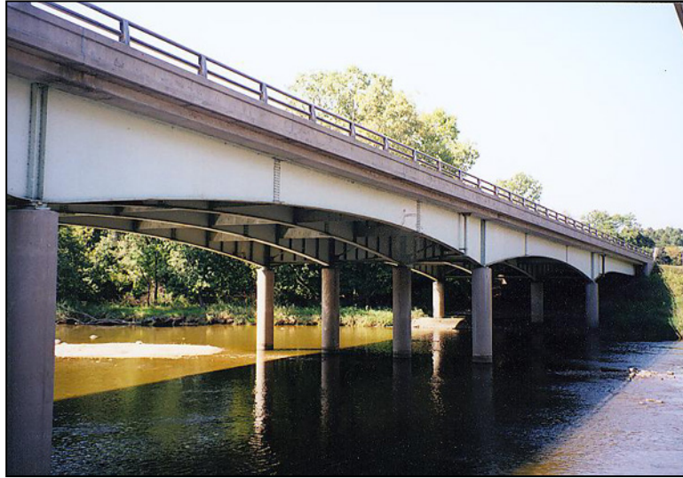
Figure 2.1.2.3-1: Continuous Spans – Steel Girders.
