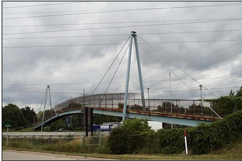
Figure 2.1.5.6-1: Cable-Stayed Pedestrian Bridge.
