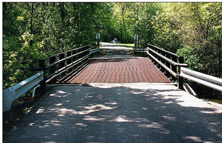
Figure 2.3.4.1-1: Open Grid Steel Deck.
