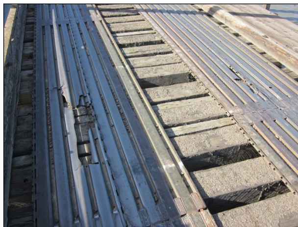
Figure 2.3.5-2: Steel Running Boards on a Timber Deck.
