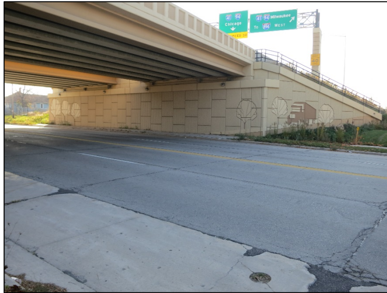
Figure 4.4.5-3: Aesthetic Treatment Form-Lined Precast Concrete Panels.
