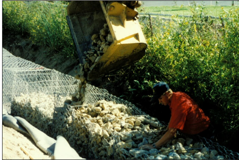
Figure 4.4.4-3: Gabion Gravity Crib Wall Under Construction.
