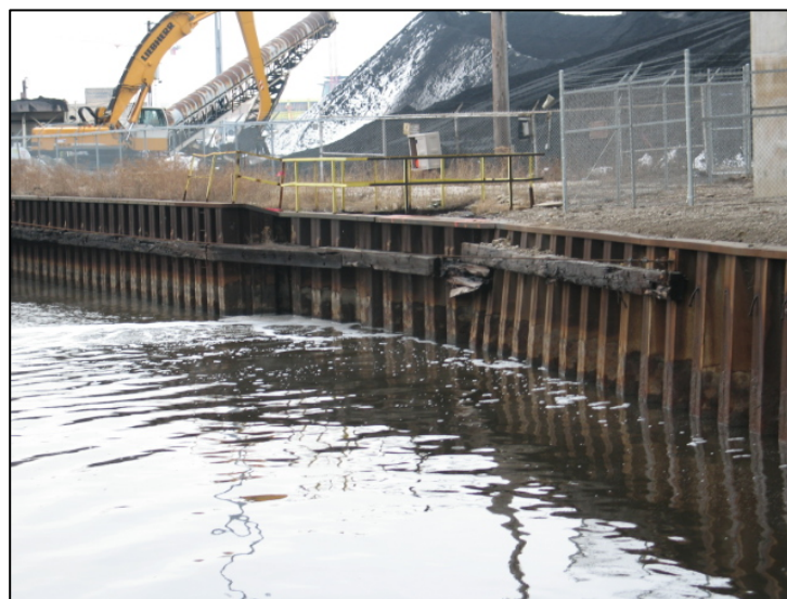
Figure 4.4.1-3: Steel Sheetpile Dockwall
