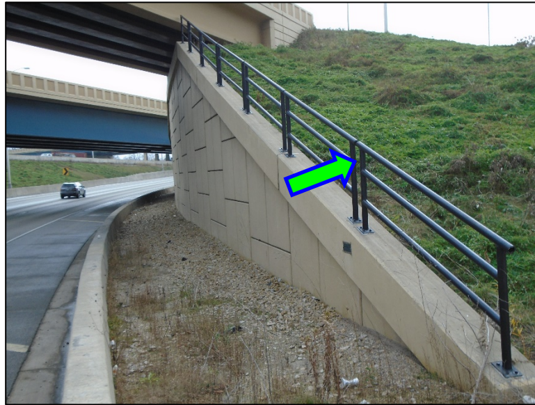
Figure 4.4.5-5: Decorative Rail atop a Horizontal Coping.
