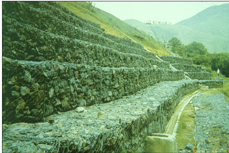
Figure 4.4.4-4: Tiered Gabion Gravity Crib Wall.
