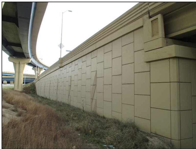
Figure 4.4.1-1: MSE "Fill" Wall
