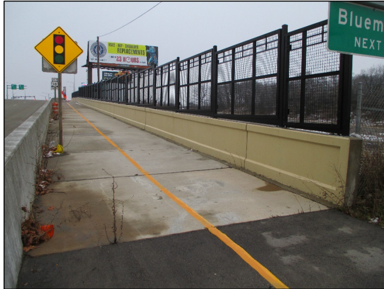
Figure 4.4.5-11: Concrete Sidewalk Along Top of Retaining Wall.
