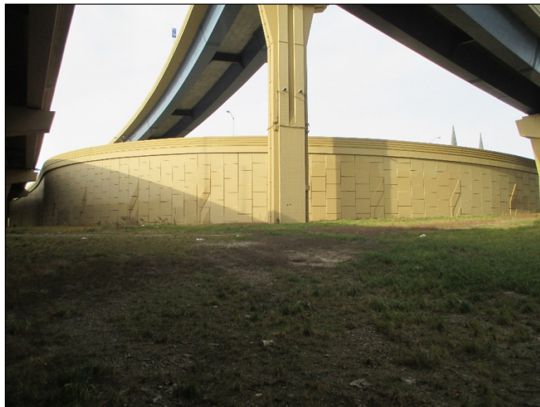
Figure 4.4.4-8: MSE Precast Concrete Panel Facing Wall.
