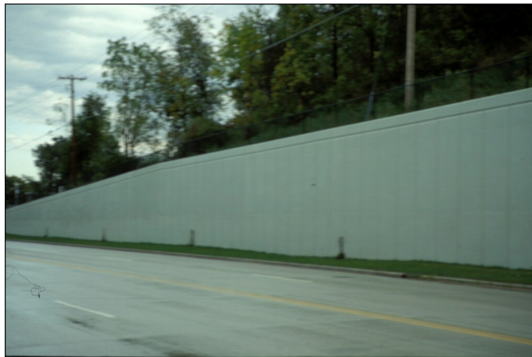
Figure 4.4.4-1: Cast-in-Place Concrete Cantilever Wall.
