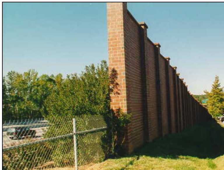
Figure 4.5.4-4: Typical Masonry Noise Barrier Wall.
