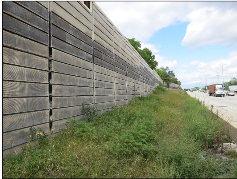
Figure 4.5.3-1: Ground Mounted Noise Wall.
