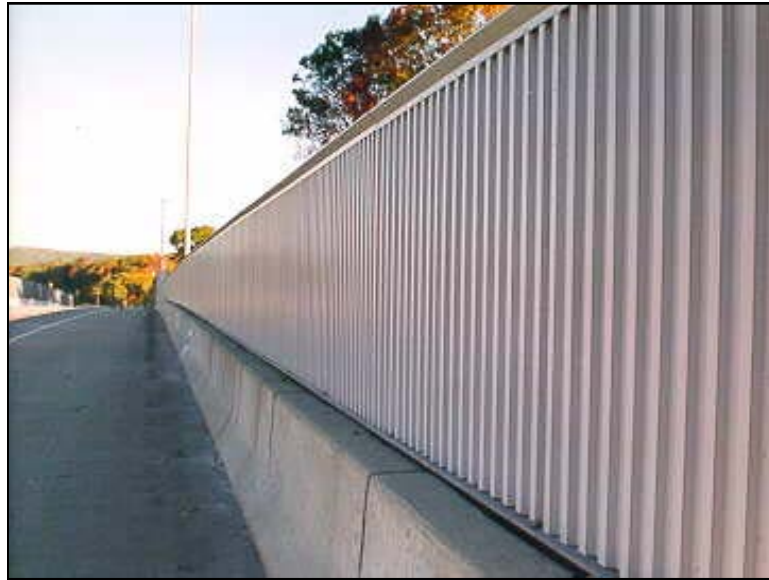
Figure 4.5.4-11: Steel Noise Barrier Wall.
