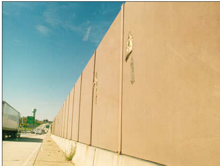
Figure 4.5.1-6: Precast Concrete Noise Barrier Wall Mounted on Concrete Vehicular Crash Barrier.
