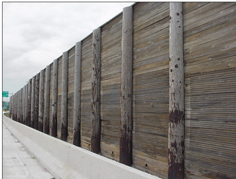
Figure 4.5.4-9: Timber Plank and Post Noise Barrier Wall.
