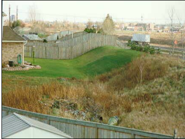
Figure 4.5.1-1: Noise Barrier Berm between Residential Buildings (Foreground) and a Roadway (Background).
