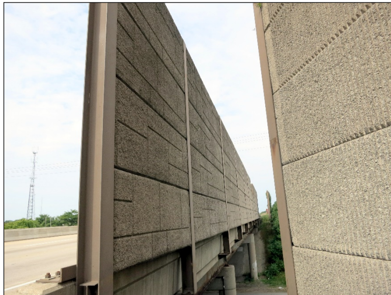
Figure 4.5.1-4: Precast Panel Noise Barrier Wall Mounted on a Bridge.
