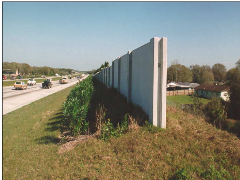
Figure 4.5.1-3: Combination Noise Barrier Berm and Wall.
