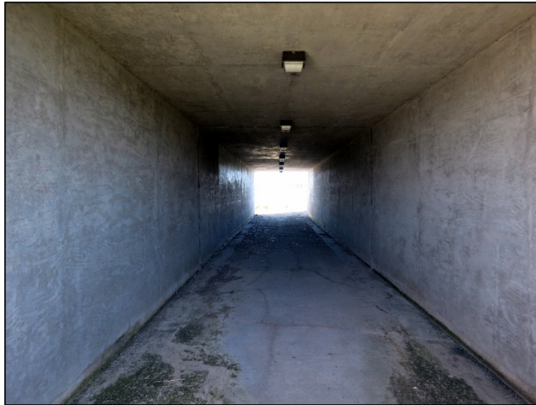
Figure 4.6.6-6: Reinforced Concrete Culvert - Condition State 1.
