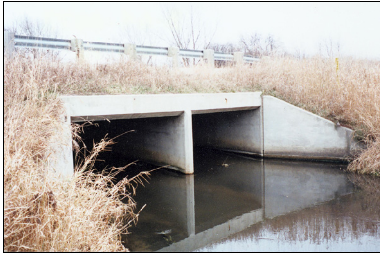
Figure 4.6.4-4: Two-cell reinforced concrete culvert.
