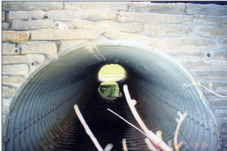
Figure 4.6.6-1: Barrel with good alignment - Condition State 1.
