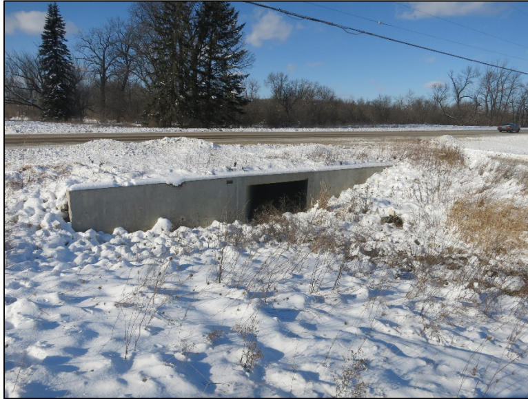
Figure 4.6.6-12: View of Integral Wingwalls Parallel with Roadway.
