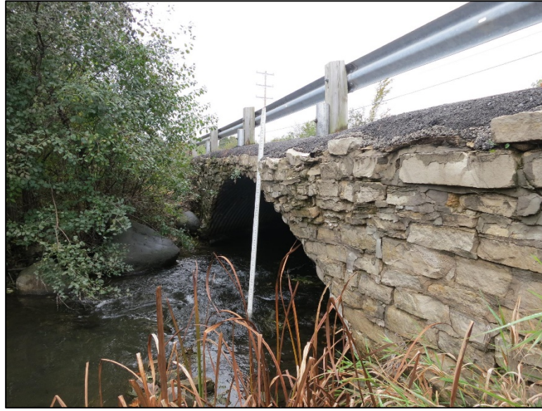
Figure 4.6.4-2: View of a corrugated steel arch culvert with masonry headwalls.
