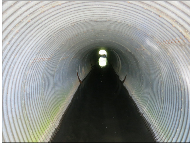
Figure 4.6.4-1: View of circular structural plate pipe culvert.
